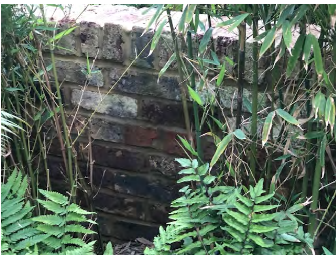
Photo 13: Rebuilt wall, Number 10 side
