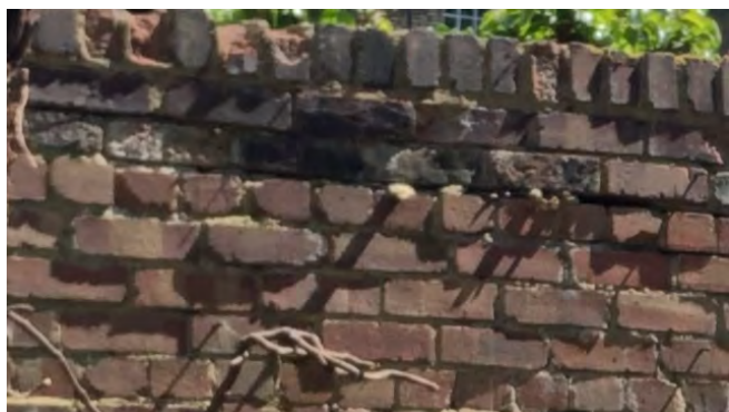
Photo 7: Quality of this section of wall
