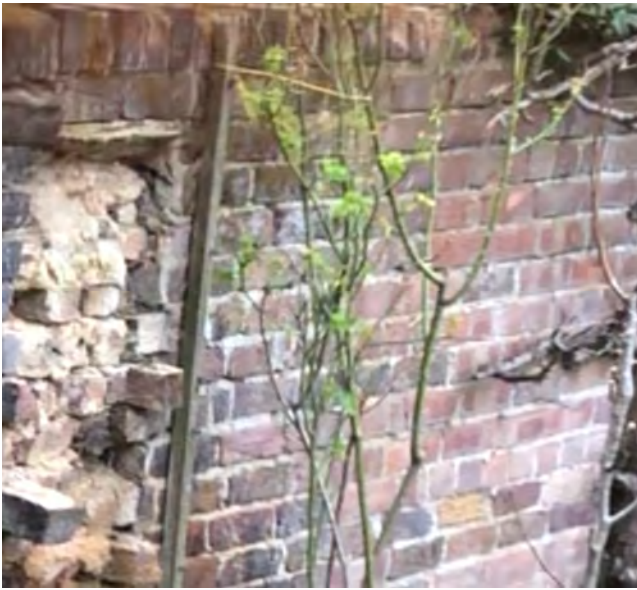
Photo 3: 2 nd pier, Number 11 side
