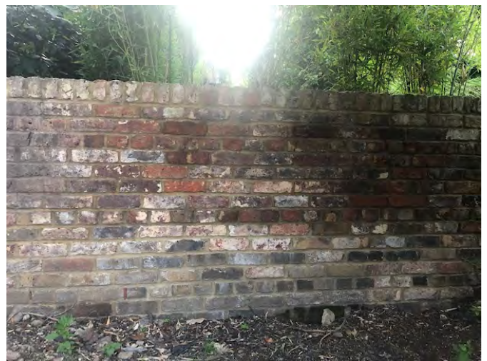
Photo 14: Rebuilt wall, Number 11 side
