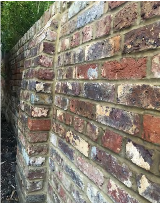
Photo 11: Rebuilt tapered 1 st pier, Number 11 side
