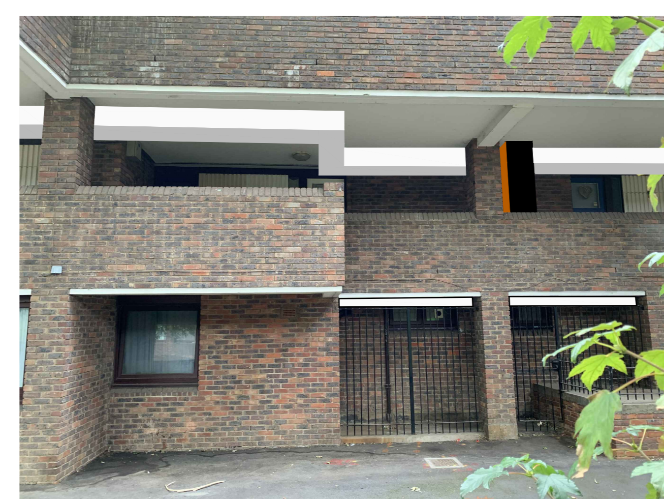
PHOTO B - GROUND & 1st FLOOR BALCONY ENCLOSURE TRANSITIONS.
