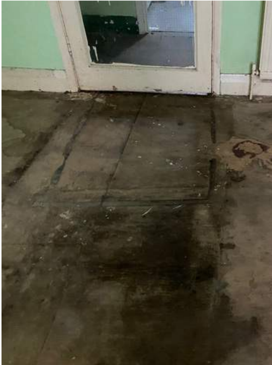
Floor showing signs of water ingress.
