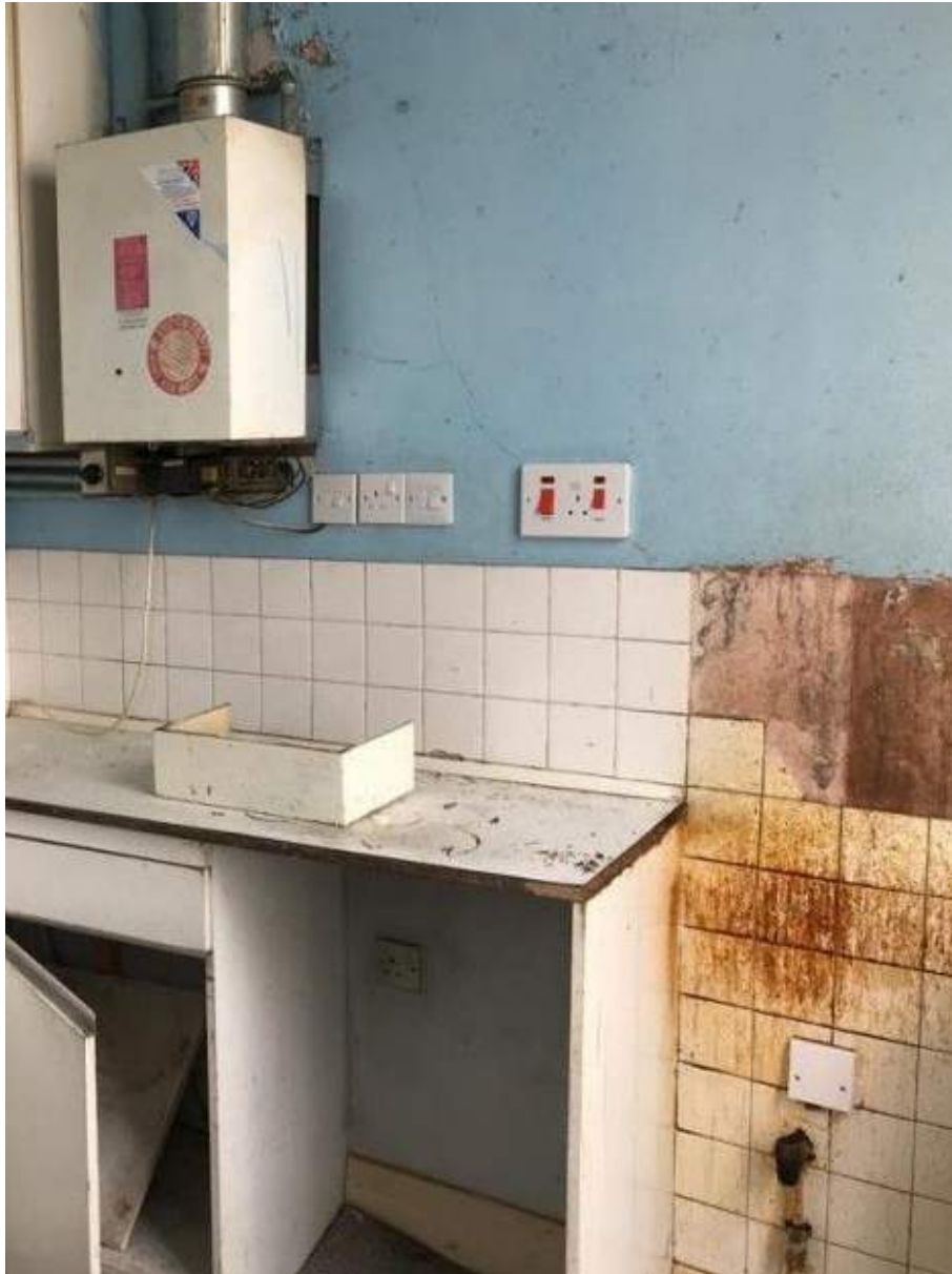
Kitchens in state of disrepair with water ingress.
