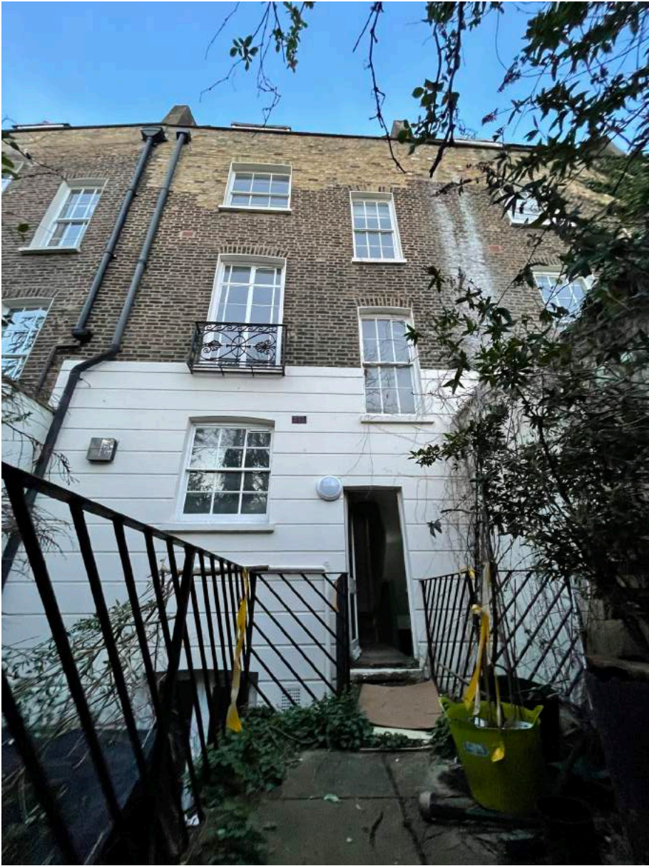
Rear elevation, showing bridge connection from ground level to garden which is not part of the original building and a more recent addition. The current levels of the basement and ground floor are inefficient and impractical, with the ground floor split between two levels as you enter the bridge connection, and the stairs leading from basement to garden being steep and non-compliant with Building Regulations.
