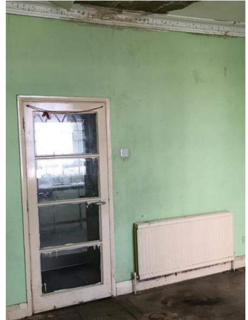
Ceilings showing water ingress from possible leakage of pipes.
