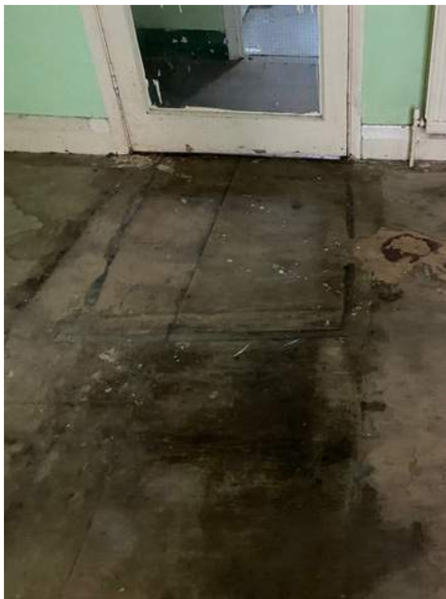
Floor showing signs of water ingress.
