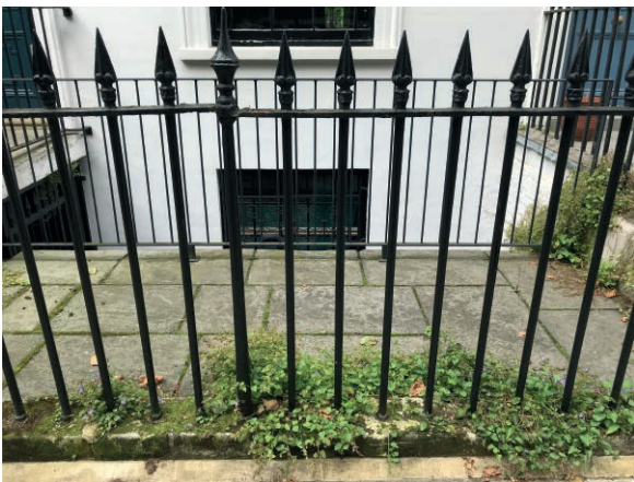
Front sandstones tiles to be replaced
