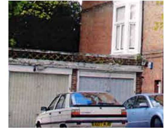
ORIGINAL HEIGHT OF BRICKWORK
