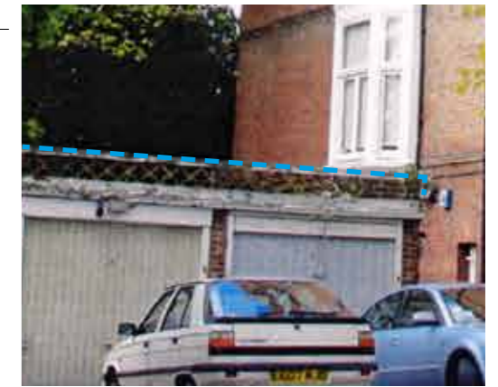
ORIGINAL HEIGHT OF BRICKWORK
