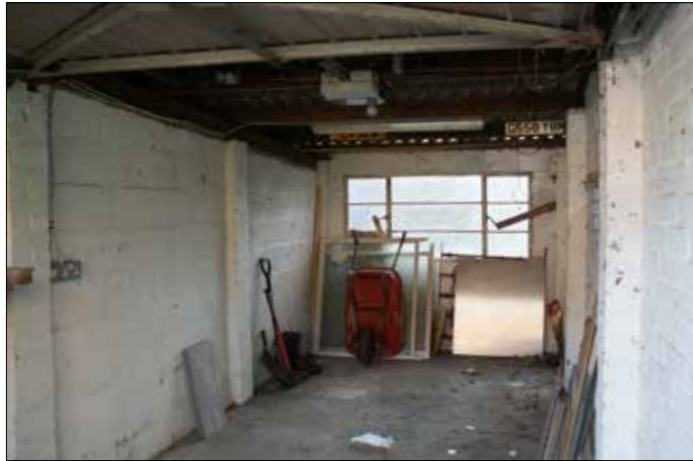
INTERNAL VIEW TO GARDEN-FACING WINDOW
