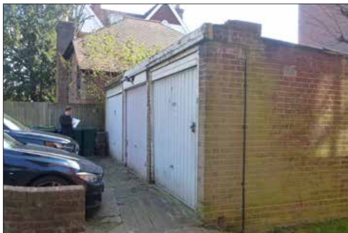
THE FRONTS OF THE GARAGES WITH CAR PARKING
