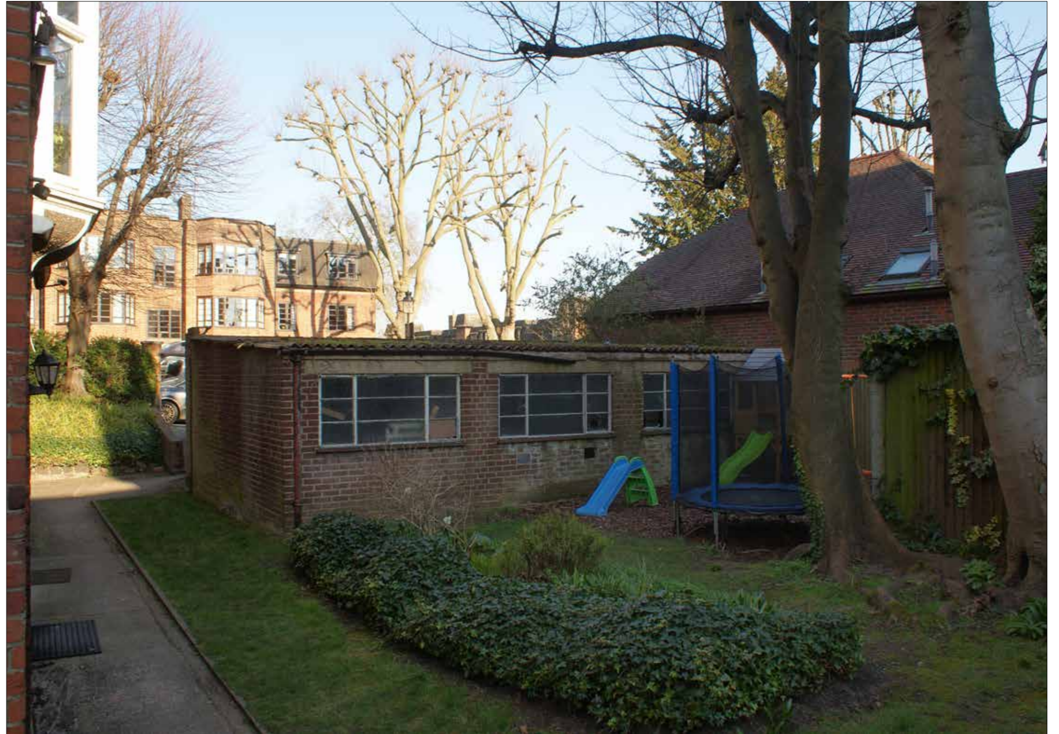
EXTERNAL VIEW OF REAR ELEVATION AND EXISTING GARDEN
