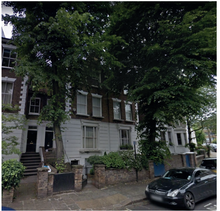
3. No. 57 Gloucester Crescent front view
