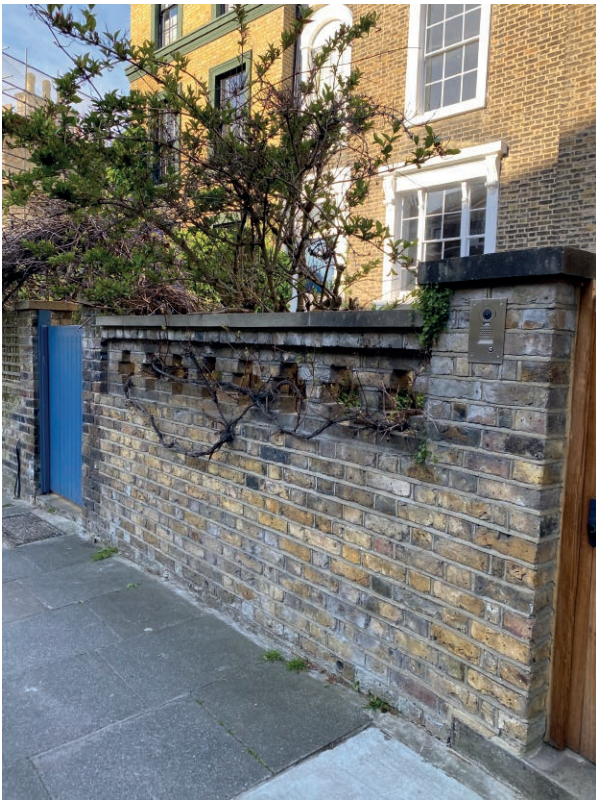
4. No. 20 Gloucester Crescent front wall detail
