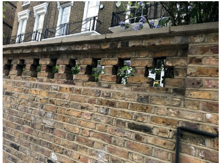
7. 27 Gloucester Crescent front wall detail
