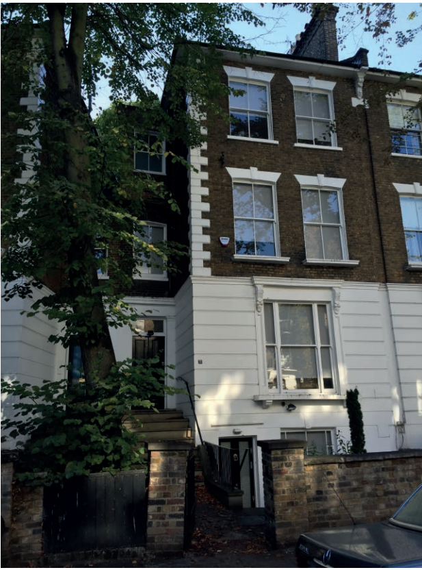
1. No. 57 Gloucester Crescent front view
