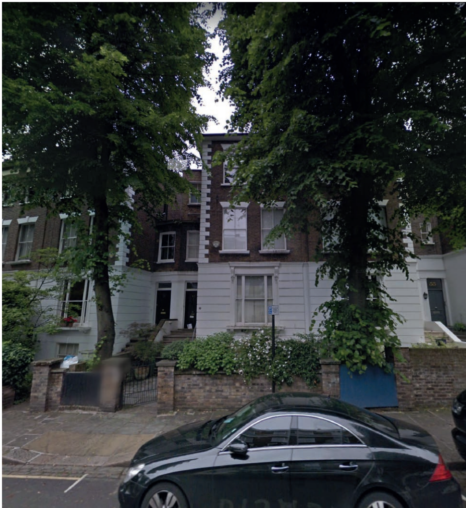
2. No. 57 Gloucester Crescent front view
