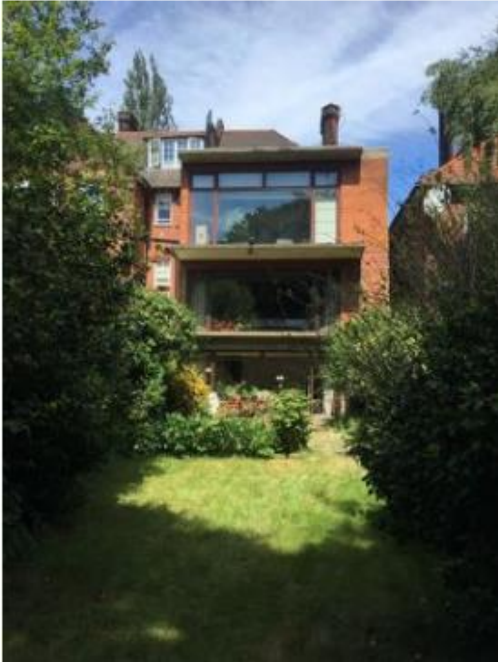
2. Rear Elevation of No. 58A Redington Road.
