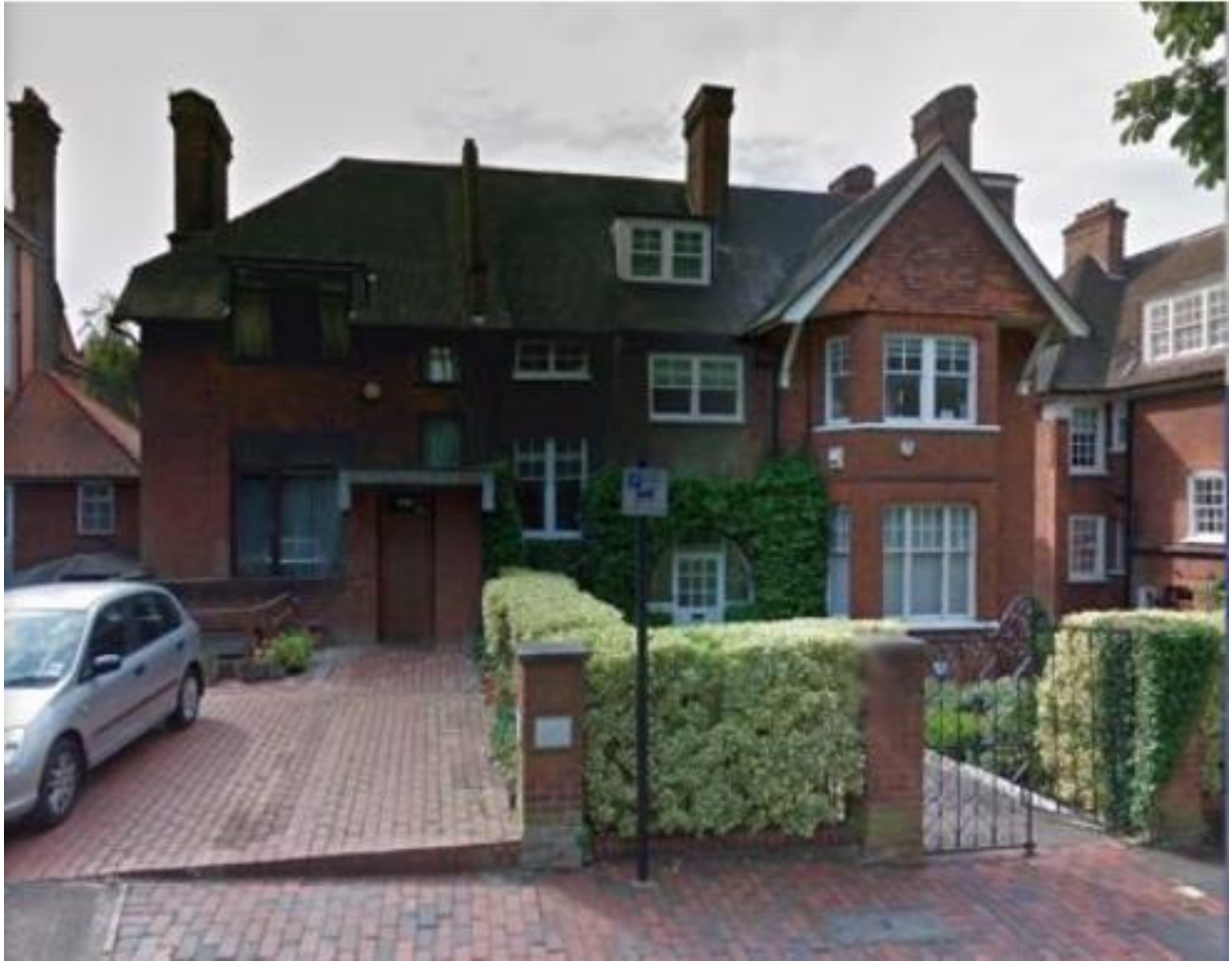
1. Front Elevation of No. 58A Redington Road.
