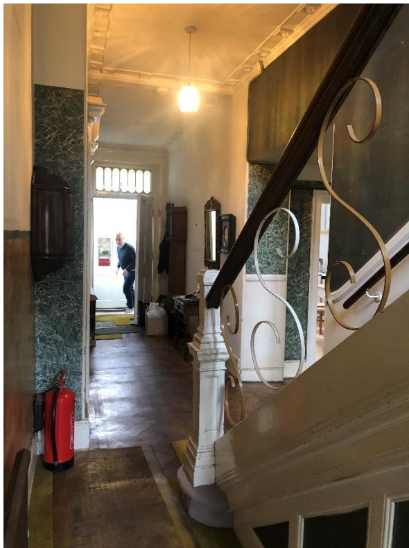
(Left) The lowest flight of the main stair with a close string, heavy newel and S-shaped metal supports to the handrail and (Right) the flight from first to second floor with a cut string and timber balusters.
