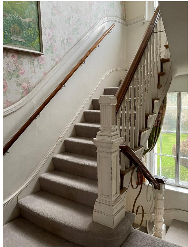
(Left) The lowest flight of the main stair with a close string, heavy newel and S-shaped metal supports to the handrail and (Right) the flight from first to second floor with a cut string and timber balusters.
