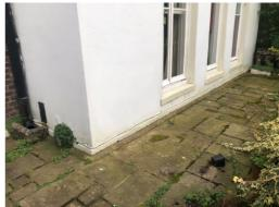
Figure 17: Fixed window to patio and bonnet blinds; Figure 18: Cills and existing York stone paving.
