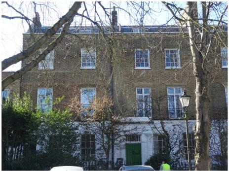
Figure 33: Front elevation casement windows to third floor, and roof safety handrail visible from street.
