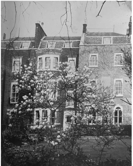
Figure 36: Historic photo of rear elevation, circa 1950s, showing original sash windows to third floor dormers.
