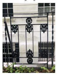
Figure 13: Painted cast iron panels on existing South Front Area, to match.
