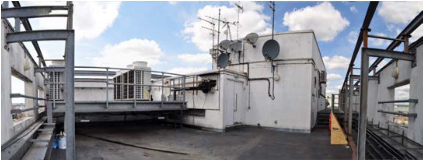
Fig. 24 - Existing Tower Roof View
