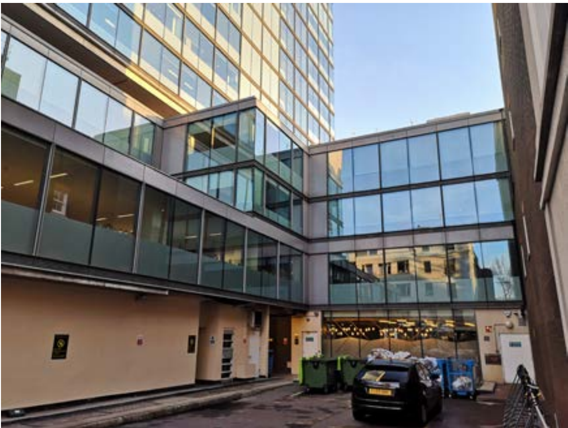
Fig. 14 - Existing Service Yard, View A
