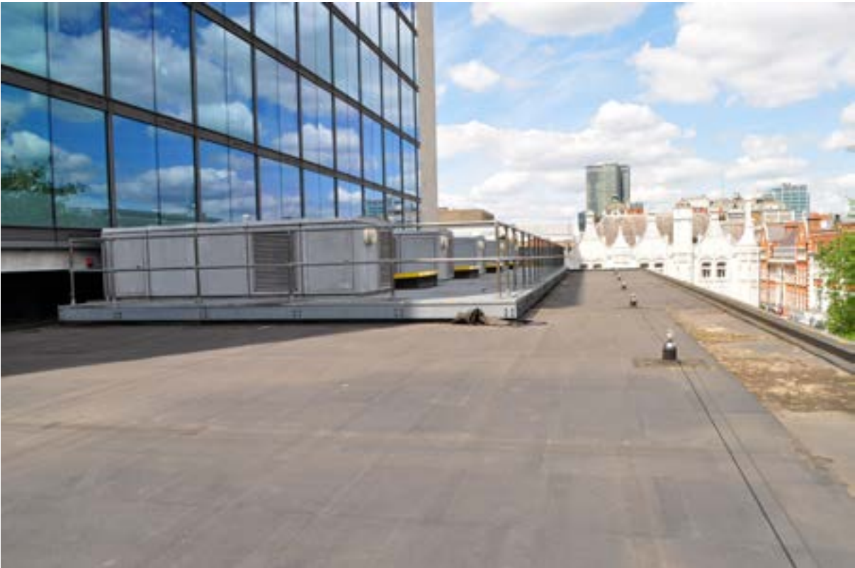
Fig. 21 - Existing Podium Roof East
