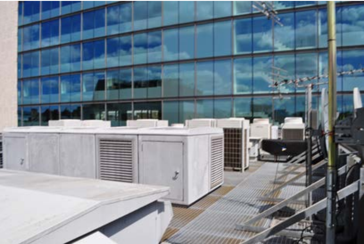
Fig. 8 - Existing, Podium Roof West Services View B
