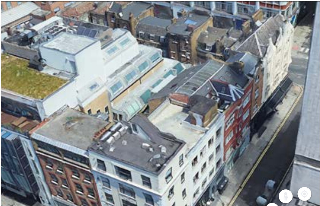
View C - Street view of opposing buildings from Windmill Street West
