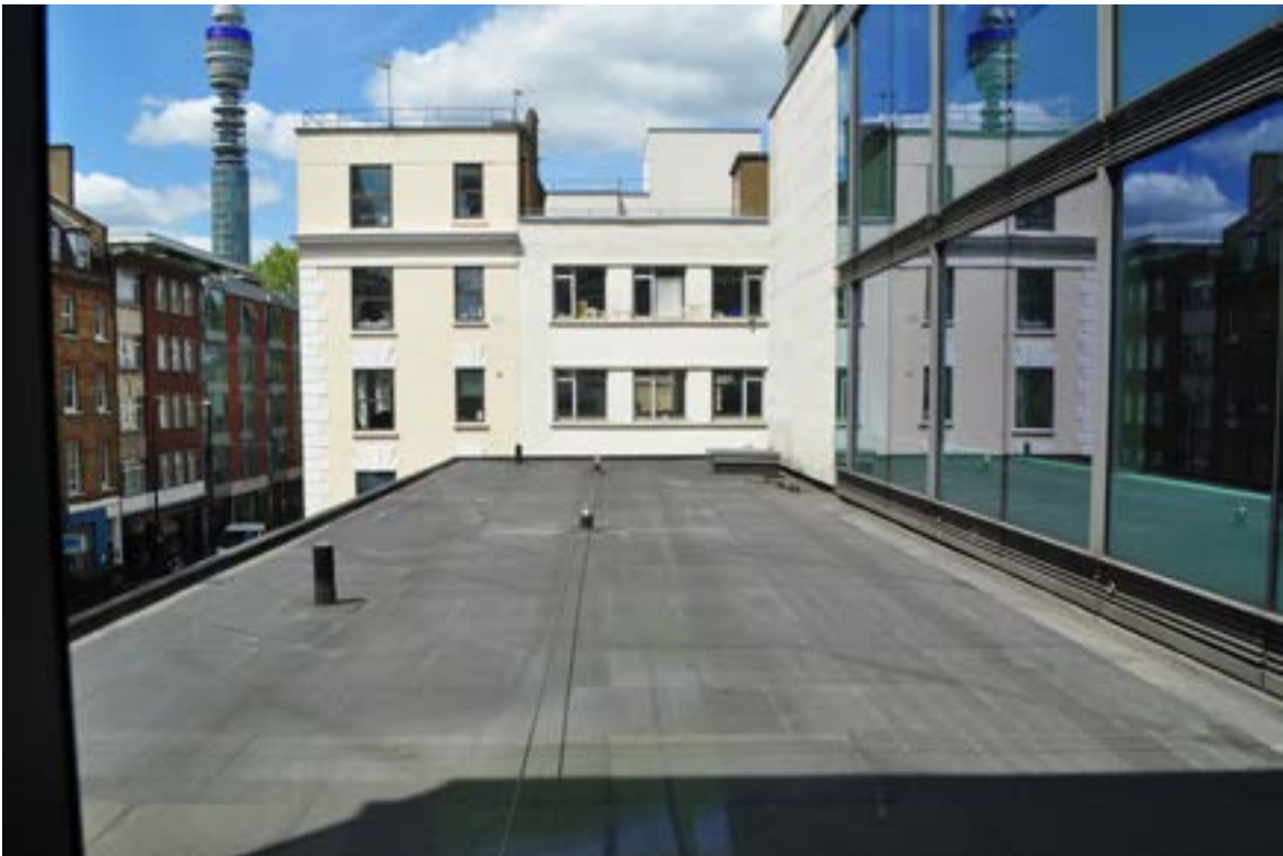
Fig. 13 - Existing Podium Second Floor Roof
