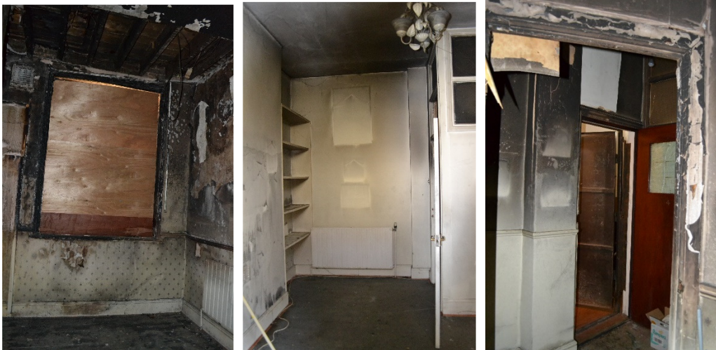
Fire damage to the sitting room and bedroom prior to fire damage.
