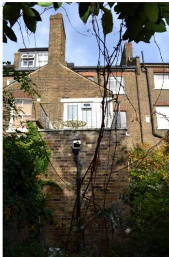
Rear elevation with dormer at No2 visible on the left
