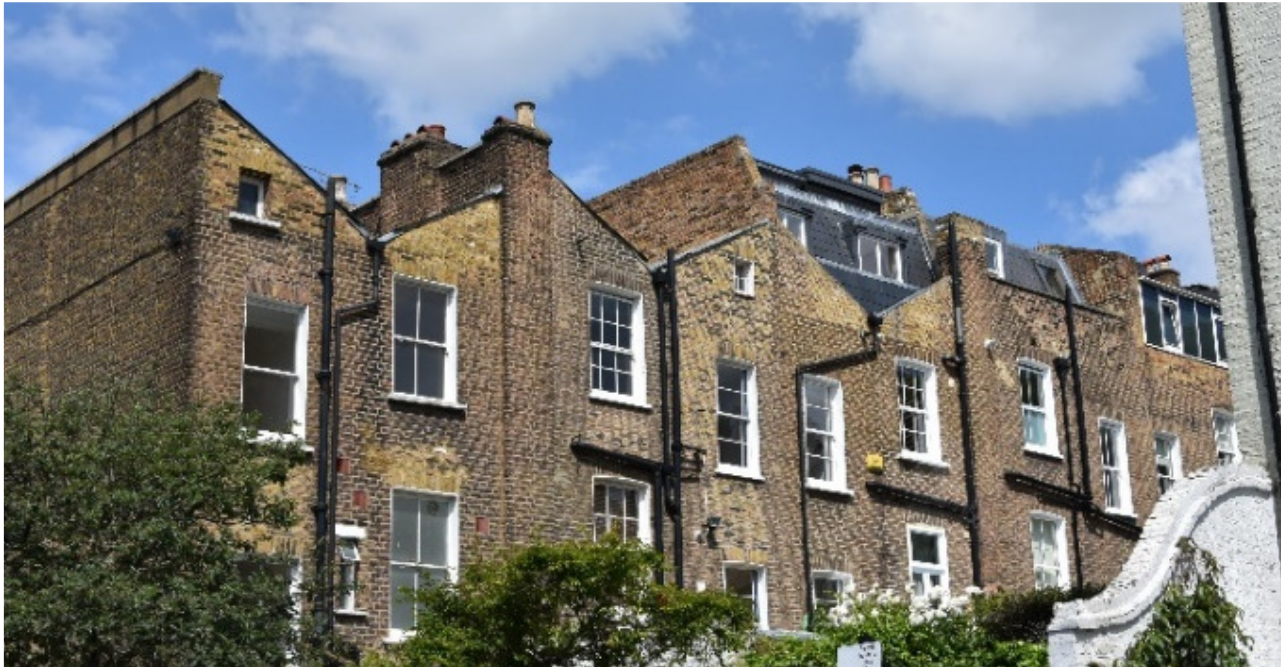
Mansard roofs at rear terrace to Leverton Street from Countess Road.
