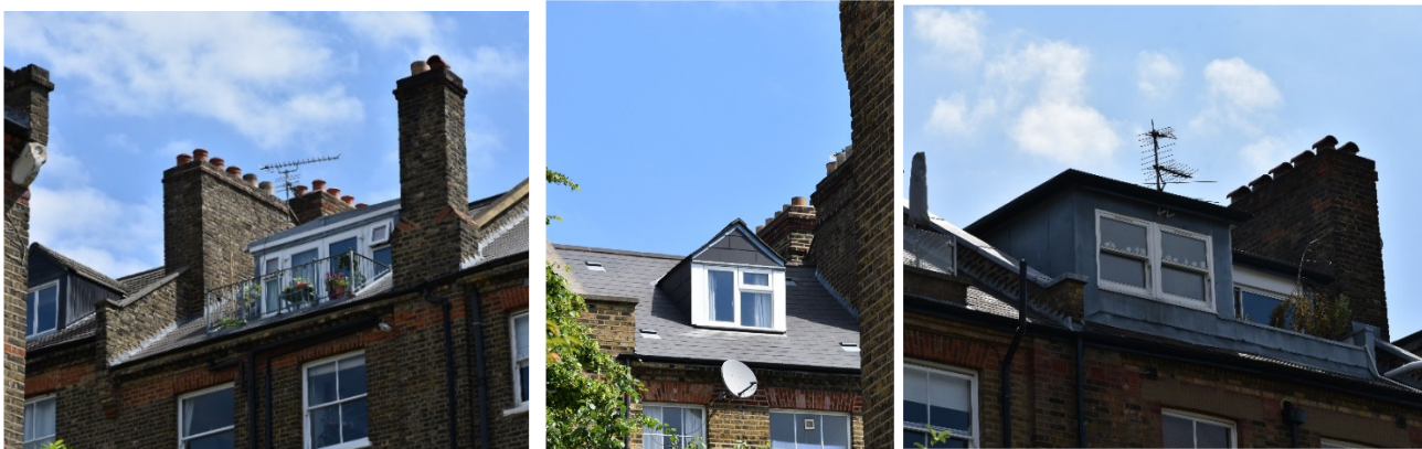
Loft conversions with in the conservation area.
