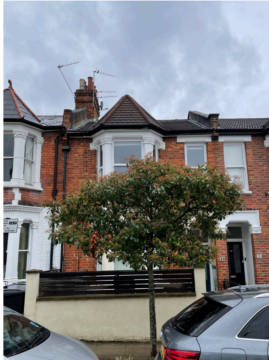
Existing front elevation of 44 Sumatra Road
