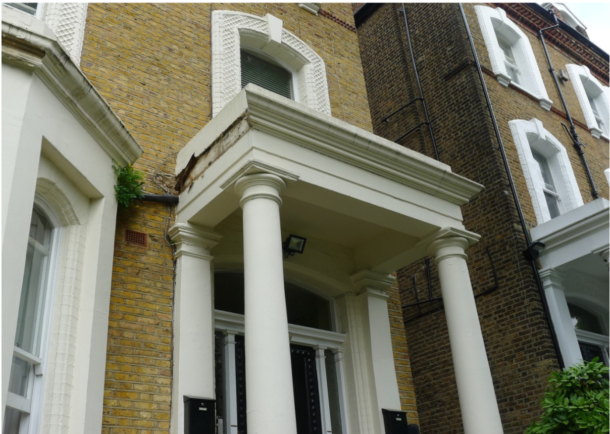
Number 47 portico and bay window cornice detail
