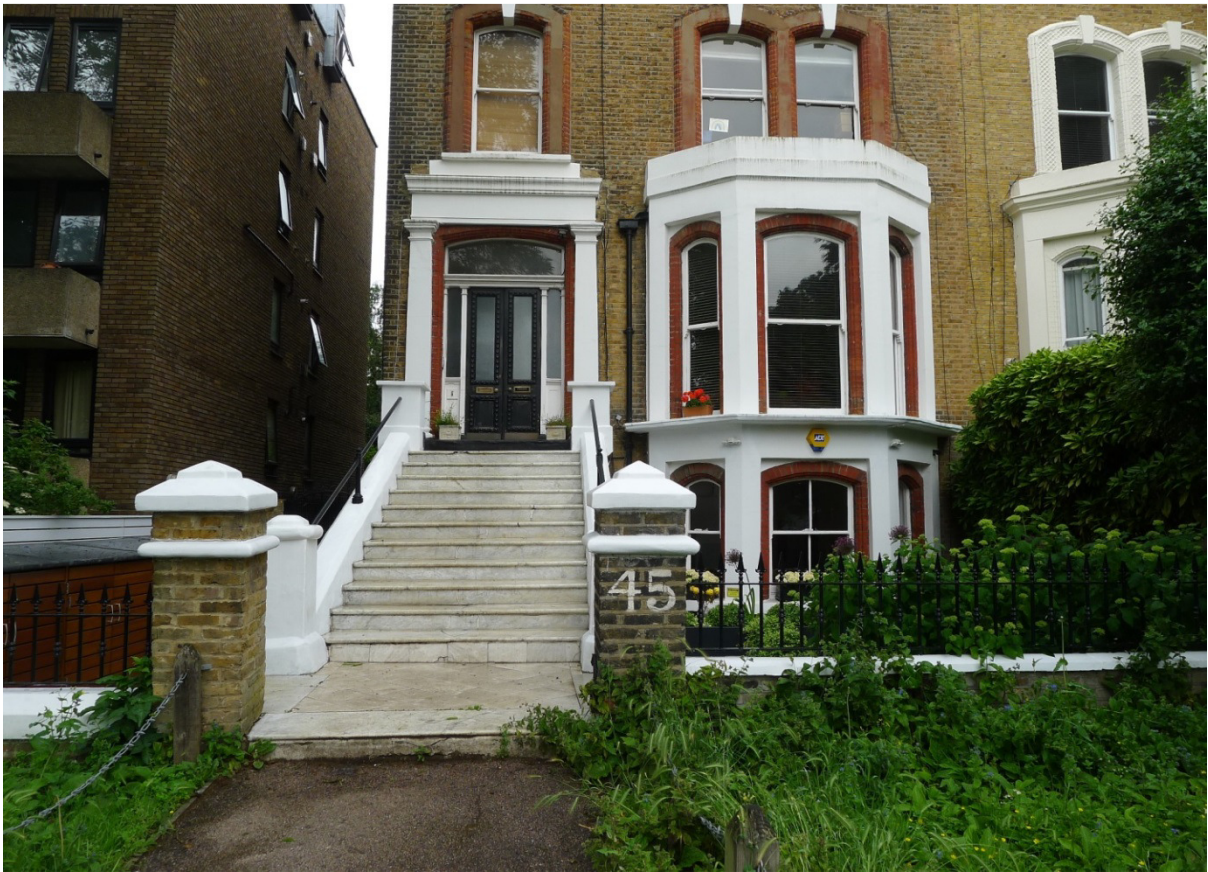
Existing portico and bay window
