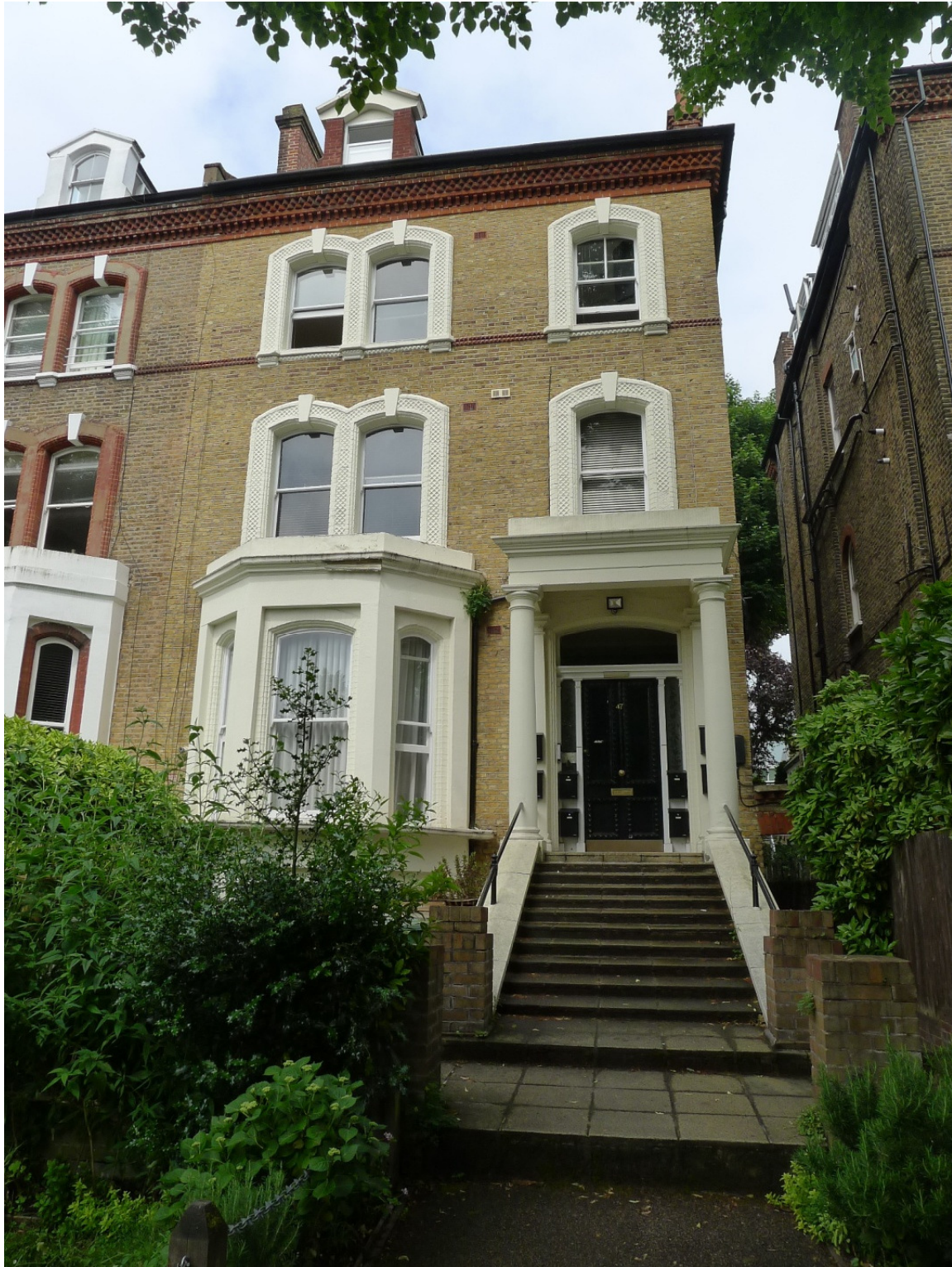
Number 47 general view of front elevation.
