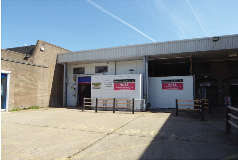
View towards factory building
