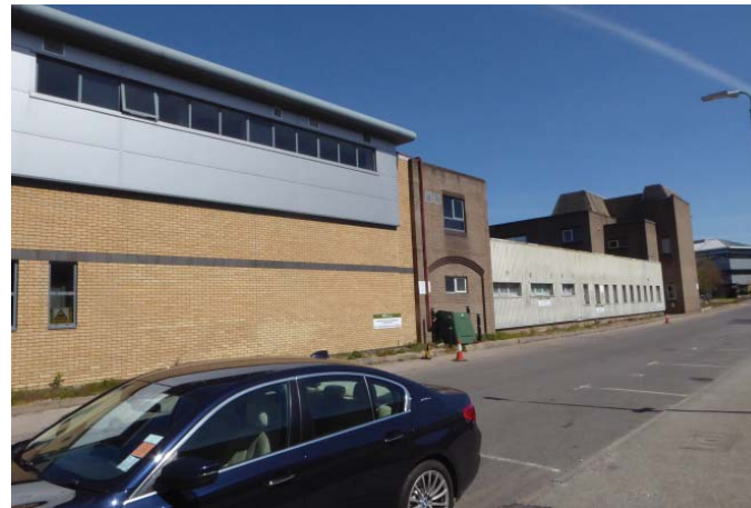
South elevation of factory building
