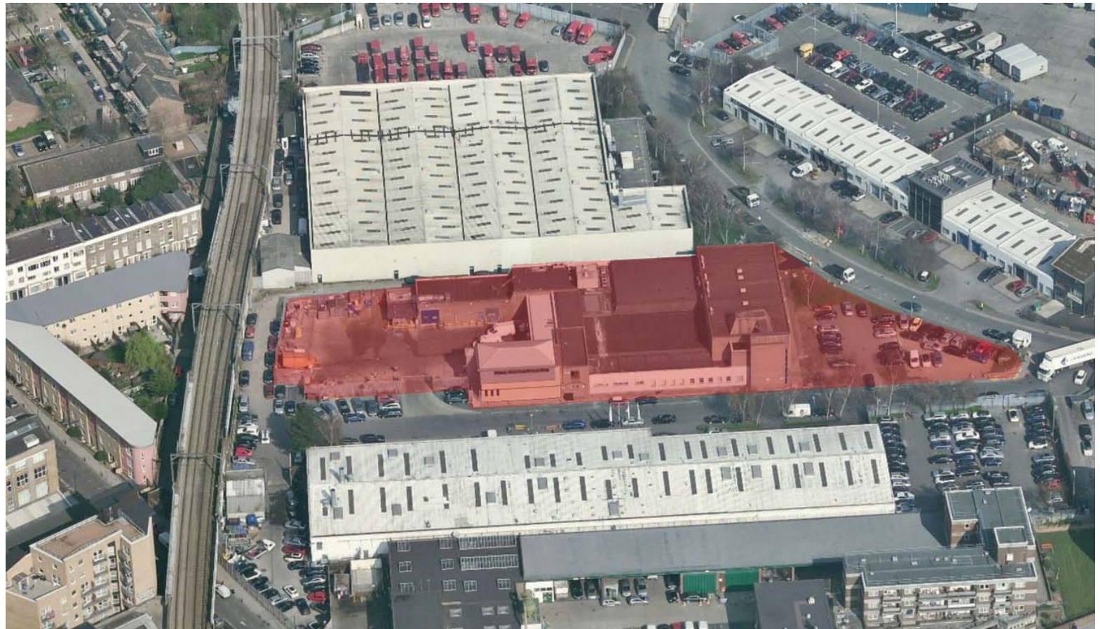
Aerial view from south (site in red)
