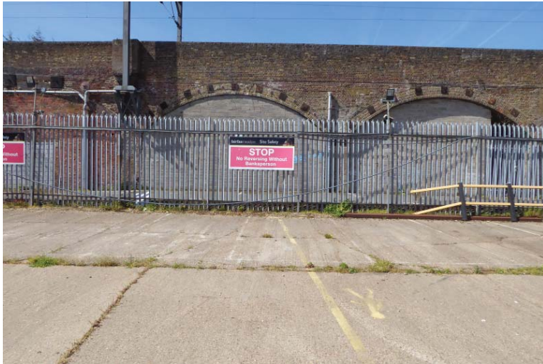
Looking towards railway line
