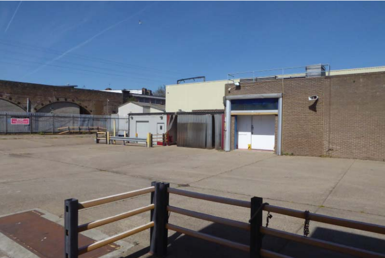
External yard looking north-west
