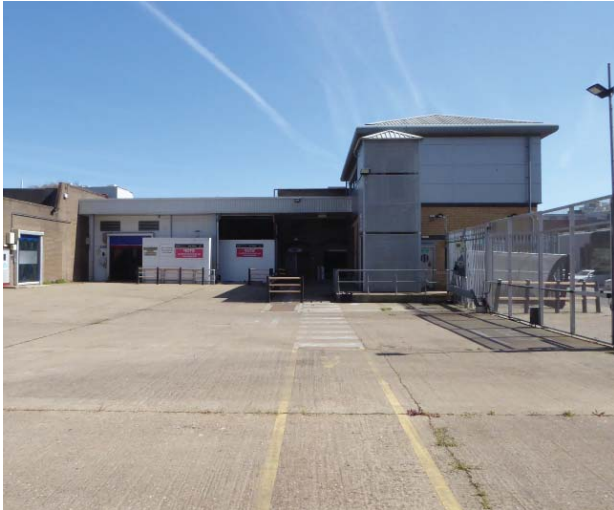
External yard looking east
