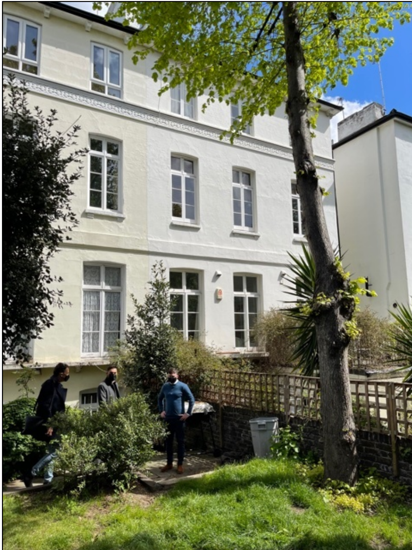
Photograph 2: Existing rear elevation with T1 visible to right
