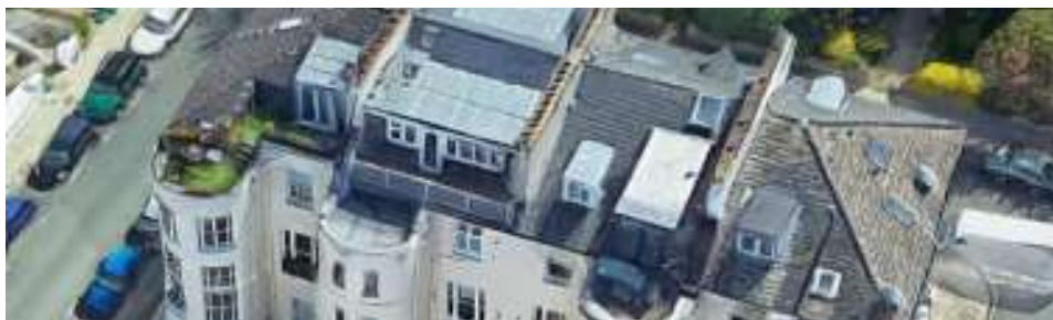
Surrounding properties have similar roof terrace dormer extensions. See section 3.0
