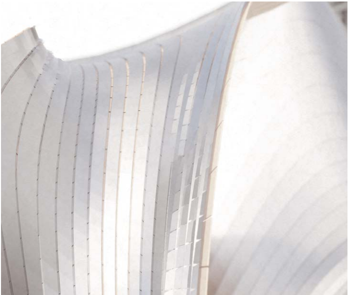
External Material - Curved Aluminium Panels
