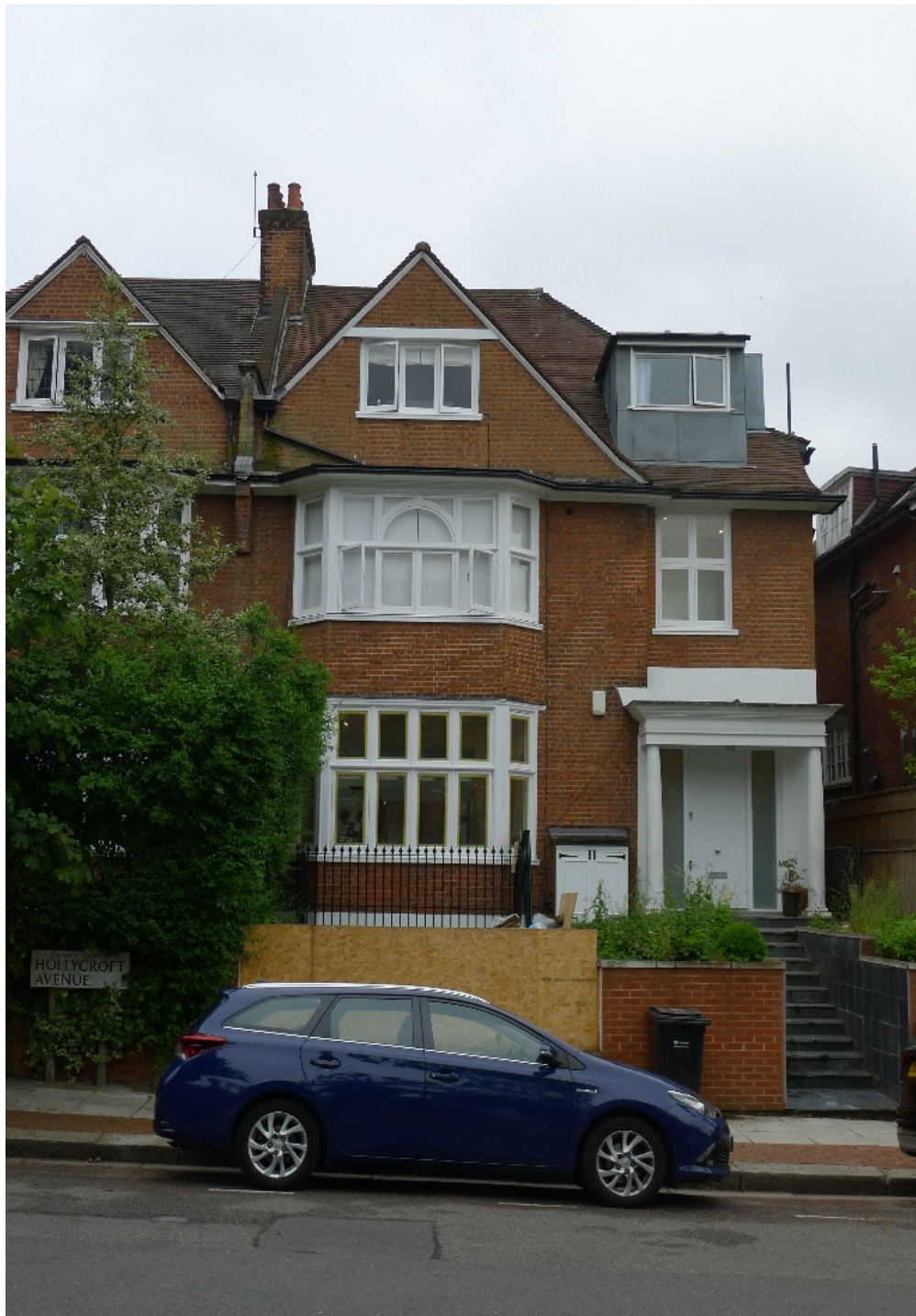
Front elevation of number 36 facing Hollycroft Avenue
