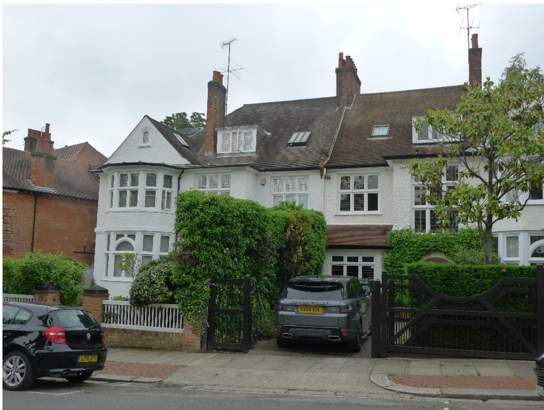
17 Hollycroft Avenue conservation rooflight on gable
