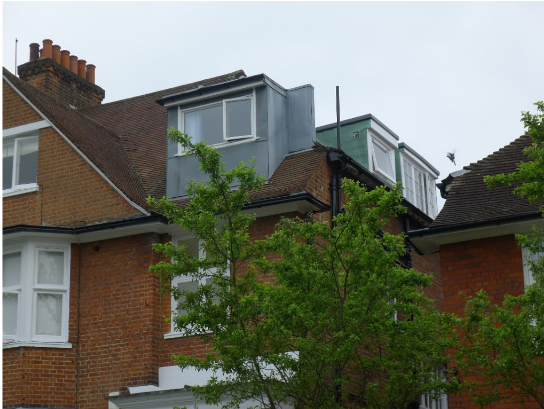
36B Hollycroft Avenue existing zinc clad dormer
