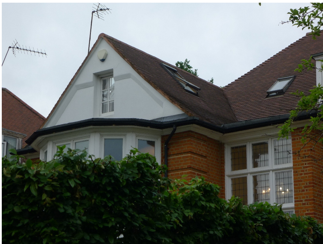
17 Hollycroft Avenue conservation rooflight on gable
