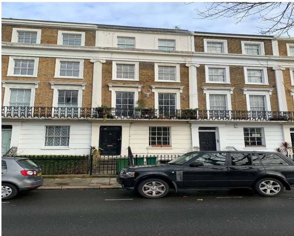
Photo 1 – Existing front elevation 36 Mornington Terrace
