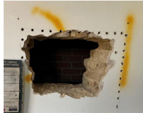
Figure 7 - Opening up works
