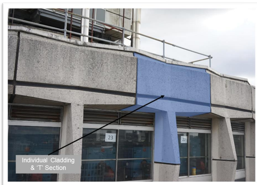
Figure 3: Existing T Sections Around 16 th Floor Slab
