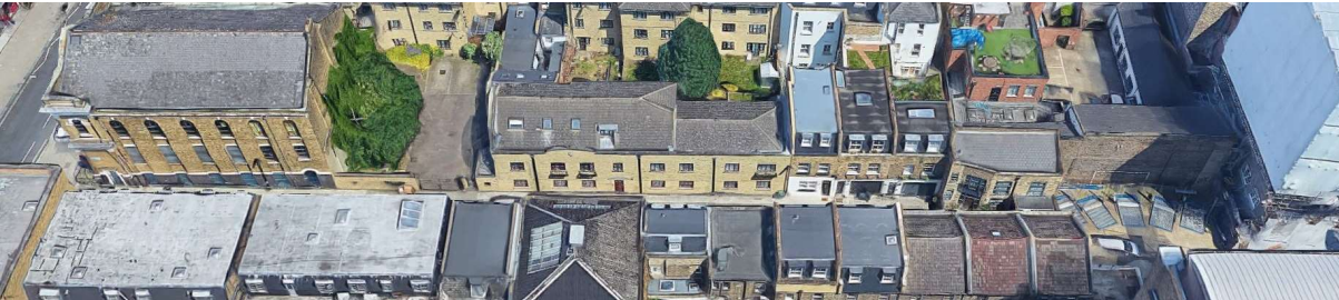
Figure 02. King's Terrace East Side
