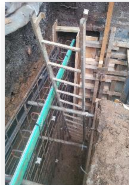
Construction of a Basement Wall by Hit-&Miss Sequence
