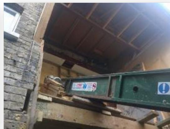
Conveyor to remove arisings
