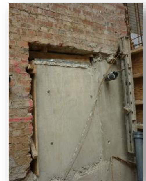
Underpinning To A Masonry Wall
