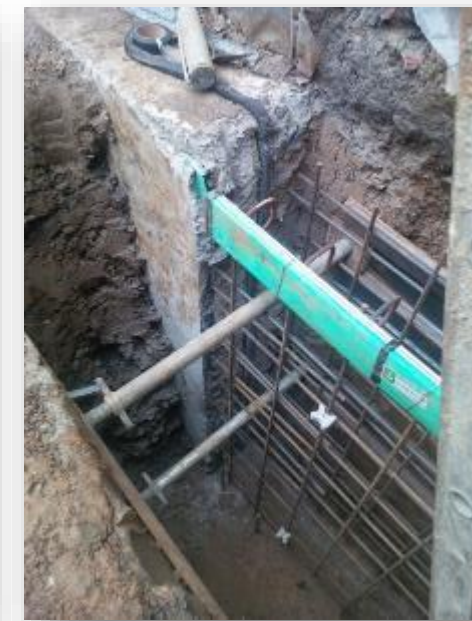
Construction of a Basement Wall by Hit-&Miss Sequence
