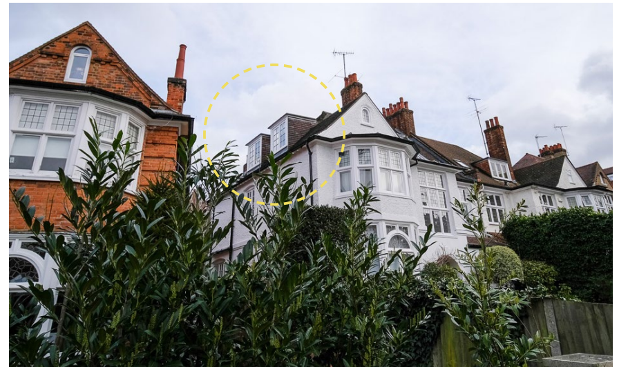
DORMER WINDOWS AT NO.17 HOLLYCROFT AVENUE (ABOVE)
