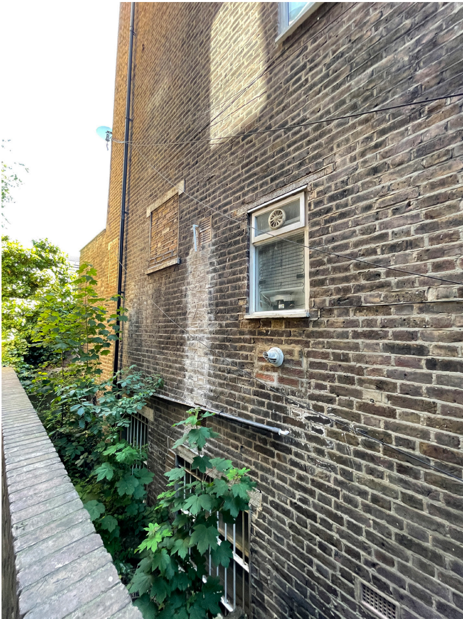
Existing side elevation of property, showing previous original window which has been infilled with brick.
