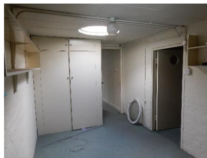
Central Attic Room
