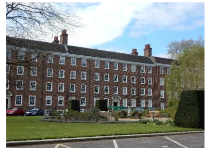
West Elevation to Gray's Inn Square (No 3 south is the 5 windows to the right of LH chimney)
