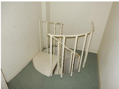
Former spiral stair access from 3 rd Floor south flat
