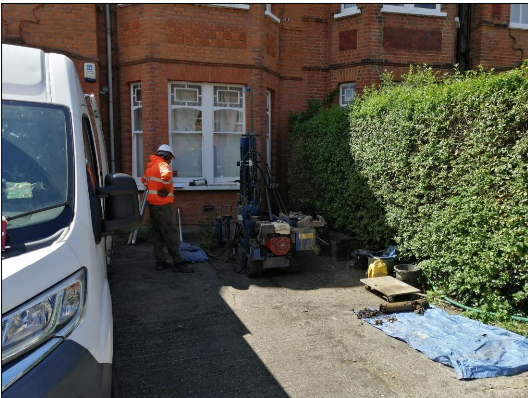
Photograph showing the Dynamic Windowless Sampling Rig in operation at BH01.
