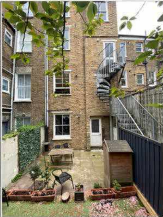
Existing Walkways steps and spiral
