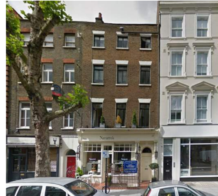
No. 67 Charlotte Street - Front View
