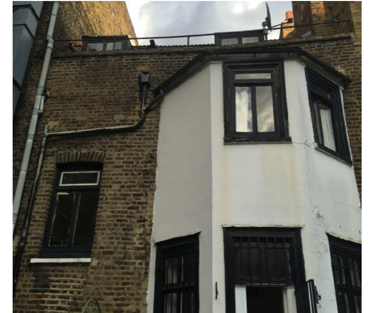
No. 67 Charlotte Street - Rear View
