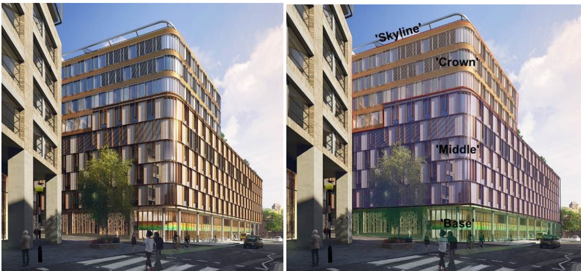
Figure 12 – View of proposed building marked up to show the three main sections of differing treatments (right image highlighted)
