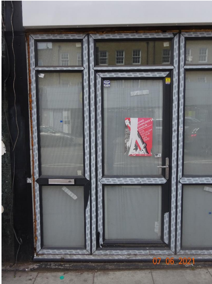
EXISTING SHOP ENTRANCE DOOR
