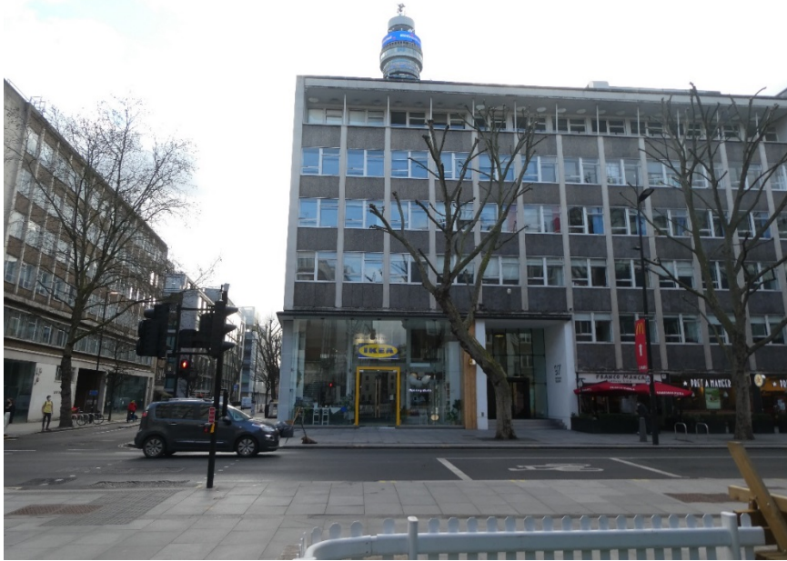
Figure 1.2 Network Building (Tottenham Court Road elevation)
