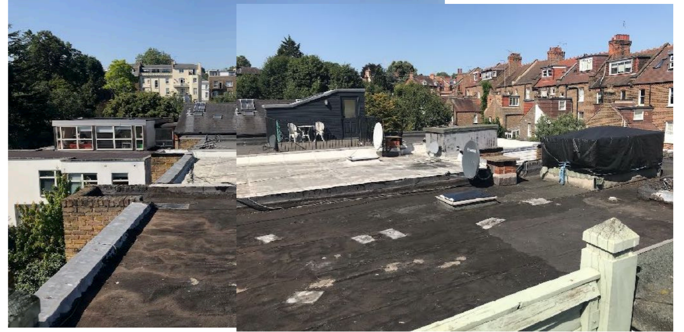
View west across roofs of 19-21 Maryon Mews
