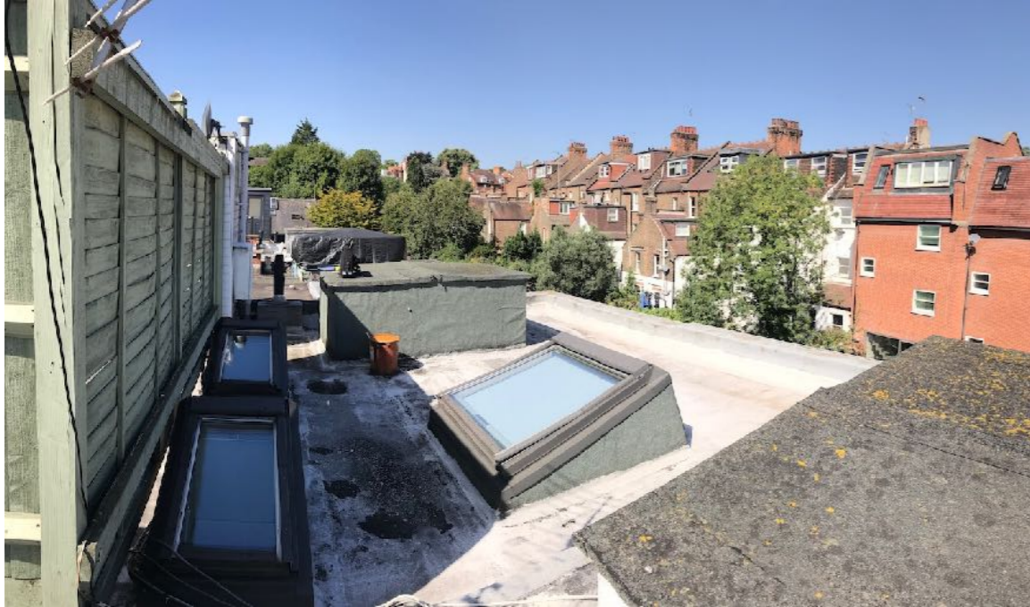
North side of Roof of 22 Maryon Mews
