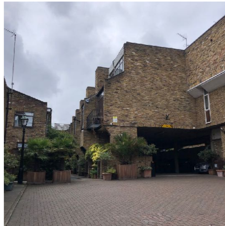
View towards nos. 19-24 from entrance courtyard
