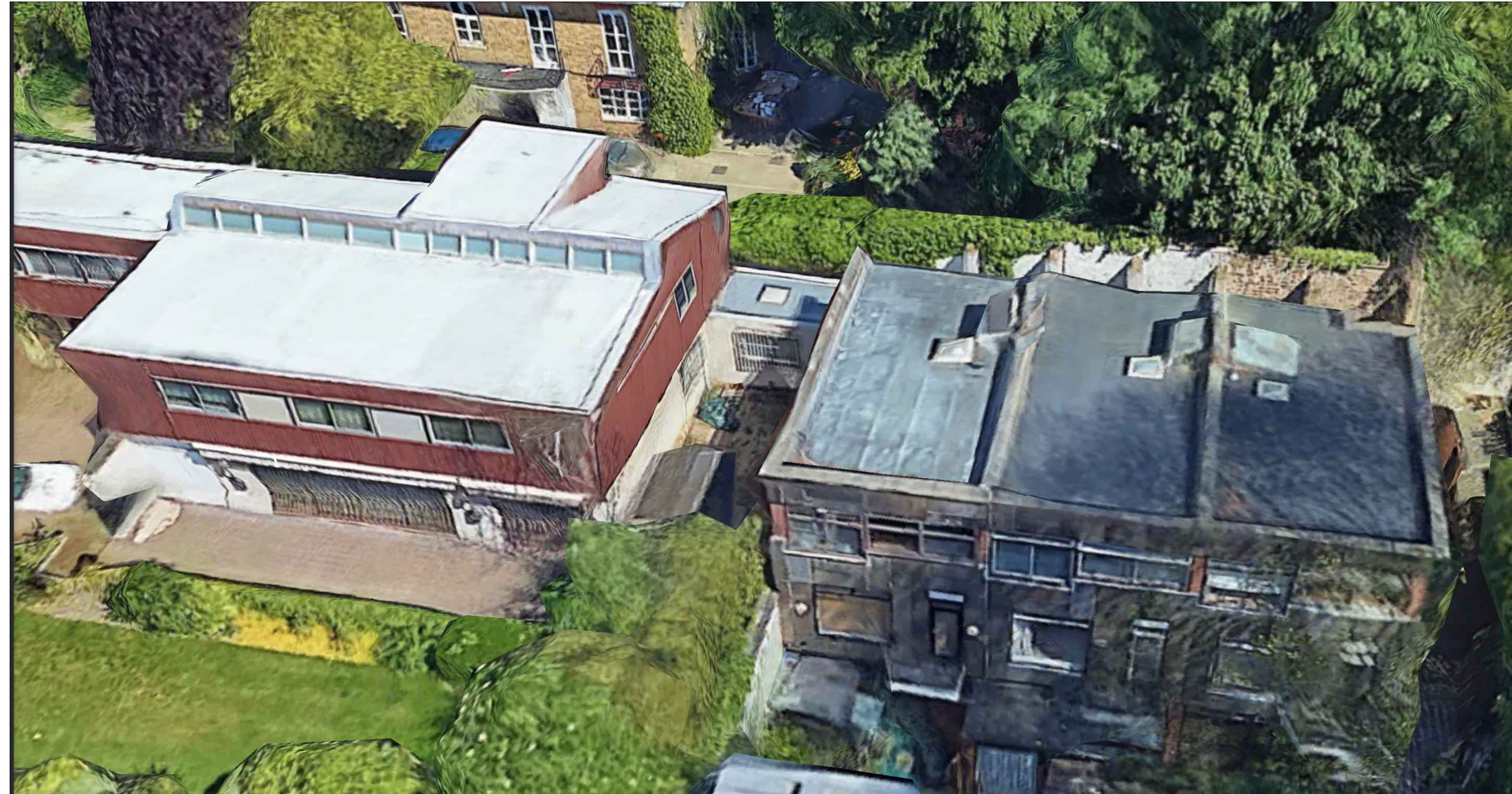
4 AERIAL PHOTO OF EXISTING ROOF TERRACE AND NEIGHBOUR AT No4 OAKHILL PARK NTS
