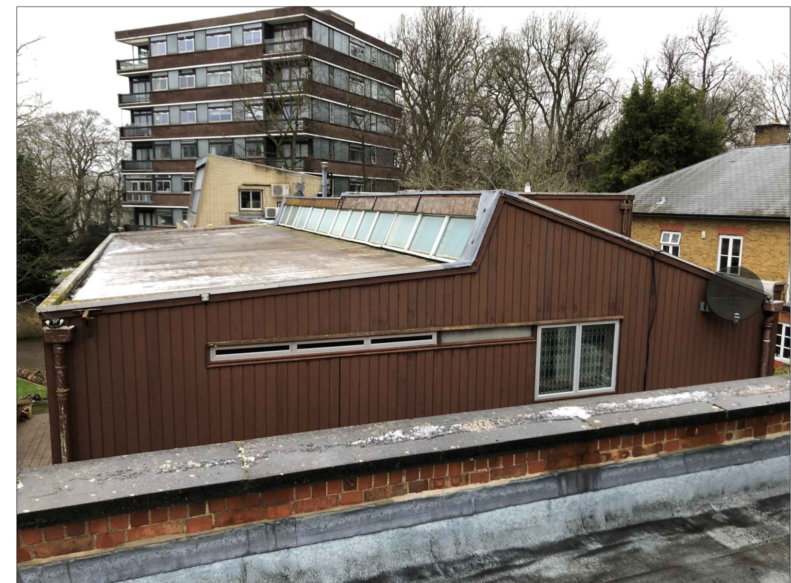
7 EXISTING VIEW FROM ROOF LOOKING WEST NTS
