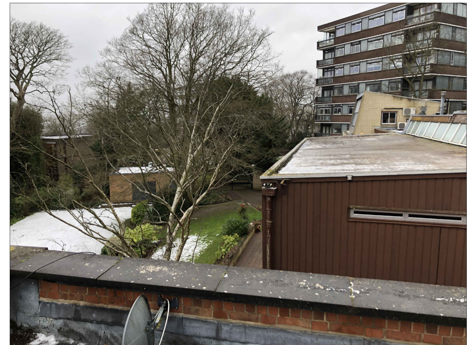
6 VIEW FROM ROOF LOOKING SOUTHWEST NTS
