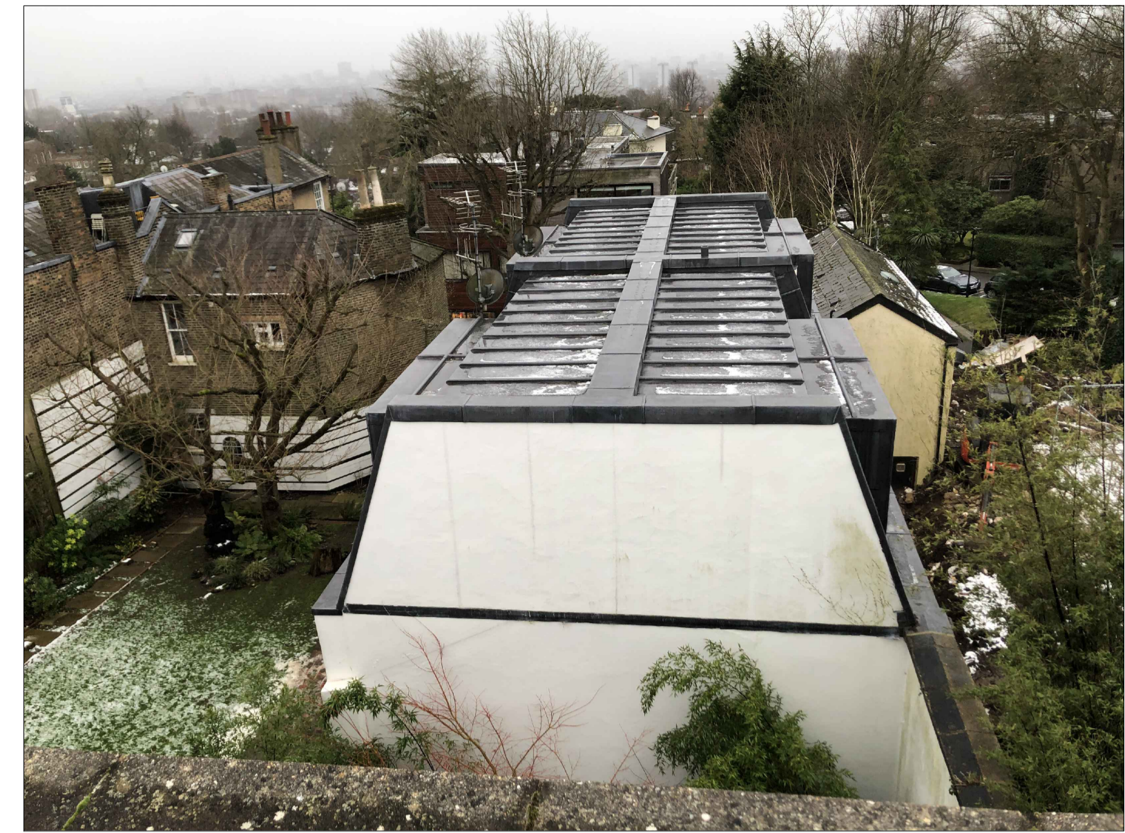
5 VIEW FROM ROOF LOOKING SOUTH NTS
