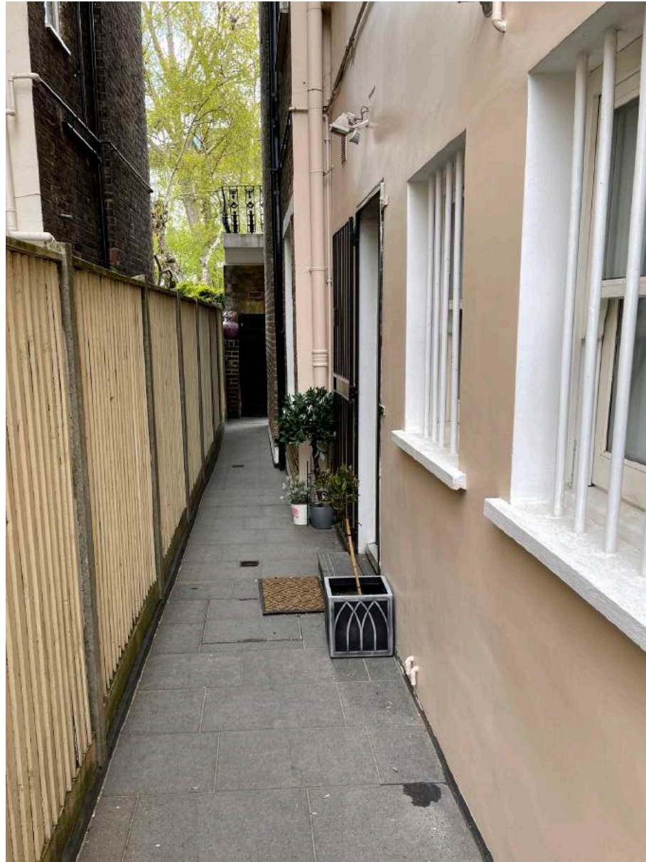
Existing side entrance as viewed entering the lower ground floor apartment.
