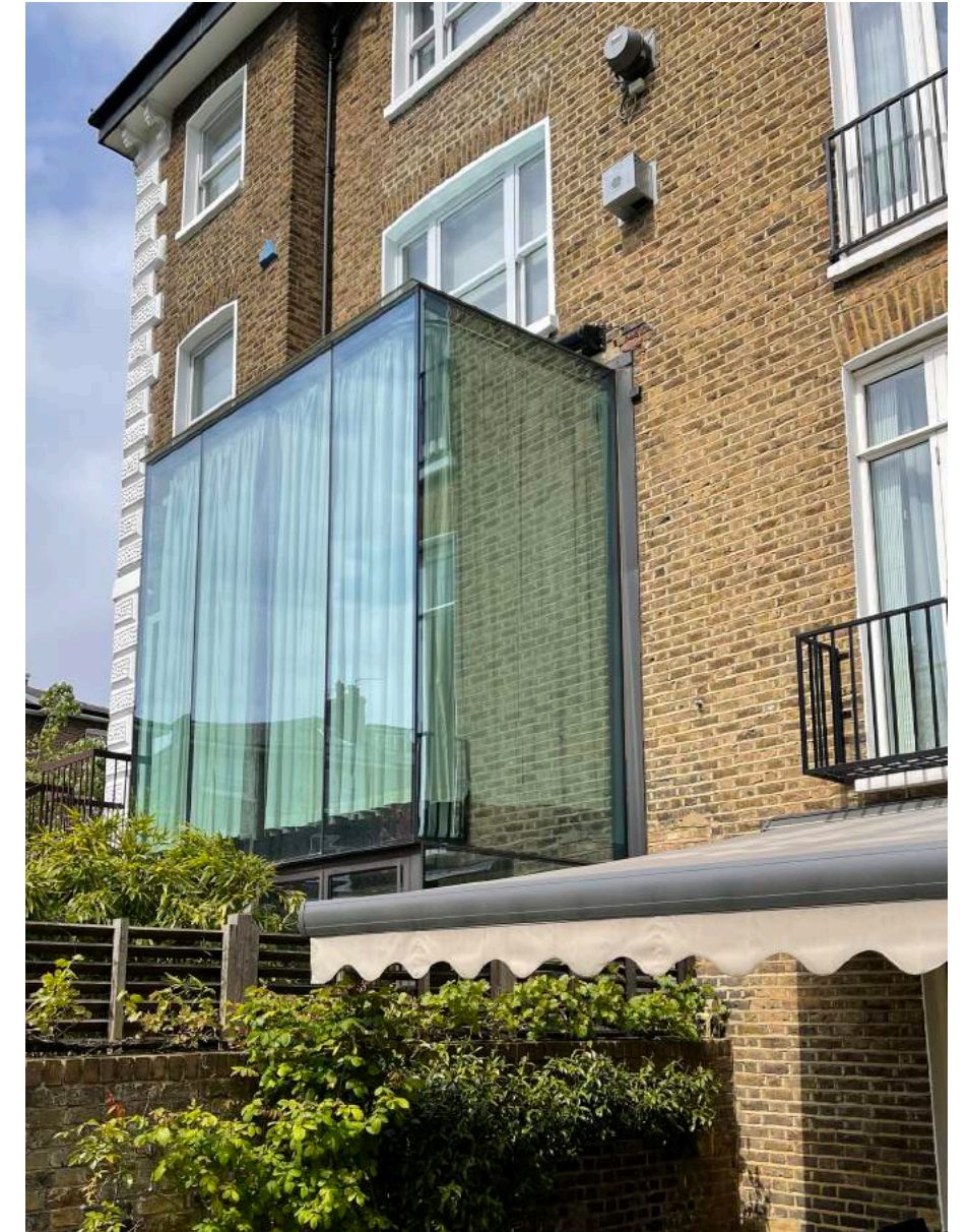
No. 1 Belsize Square double storey rear extension in a fully glazed exterior. This replaced the former lower ground and ground floor bay window which also included a ground floor terrace area.
