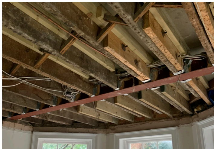
Existing Beam and Joist Strengthening
