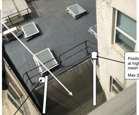
Position of fresh air inlet duct at high level, terminal with bird mesh and 90 Degree cowl,
