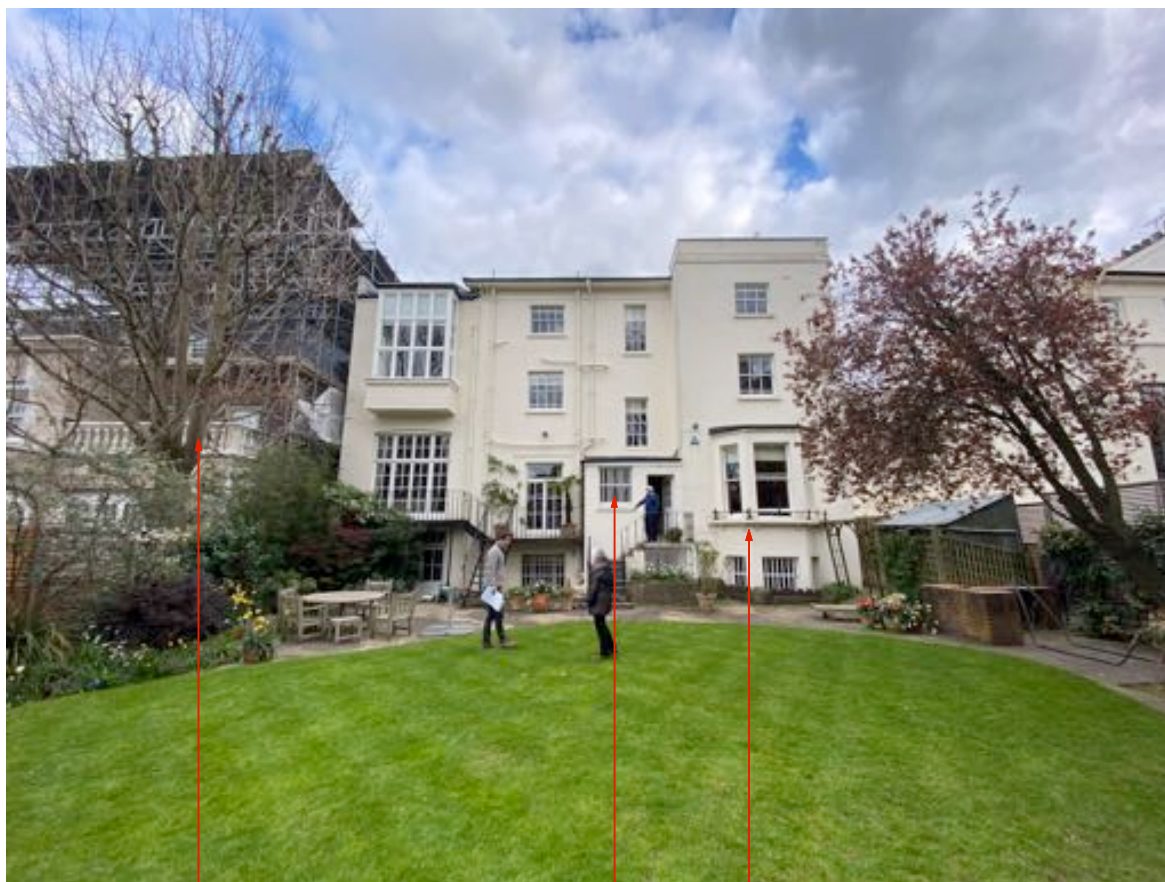
existing terrace at high level to neighbouring property
