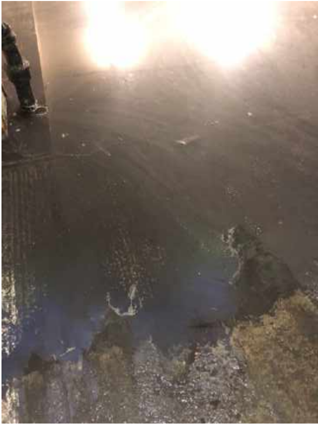
Sheen from light oils on pooled water in the basement
