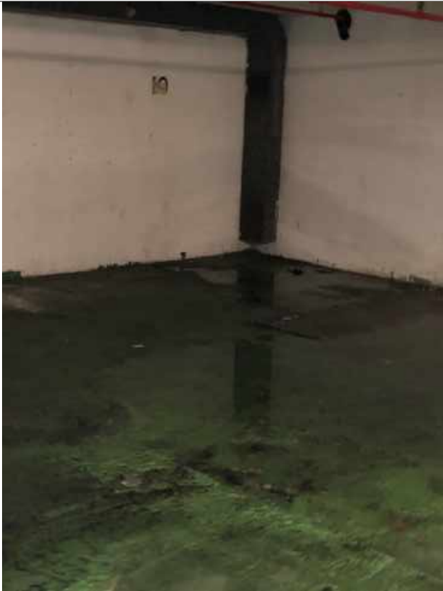
Basement flooding due to pipe malfunction
