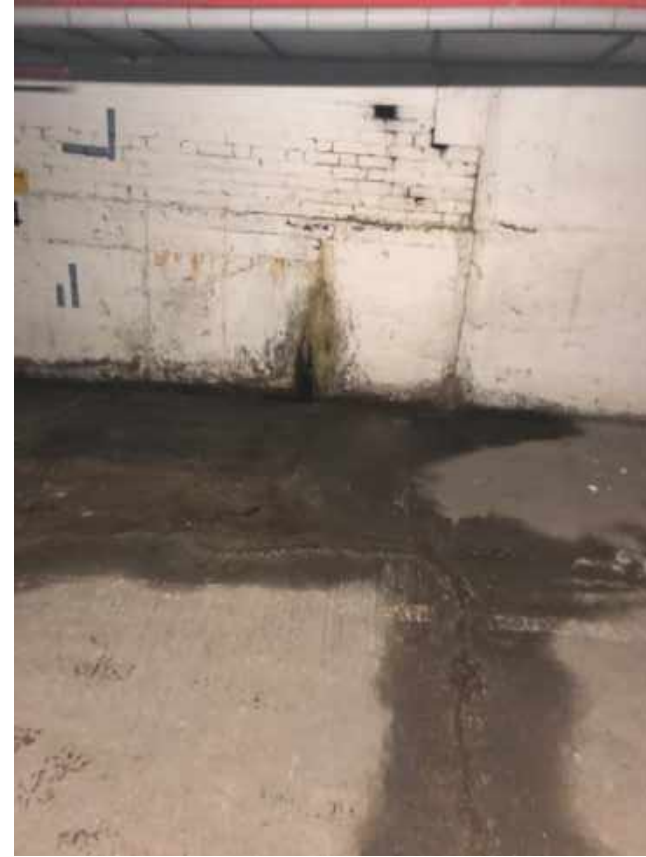
Limited cracking in the basement floor and wall with associated water seepage marks
