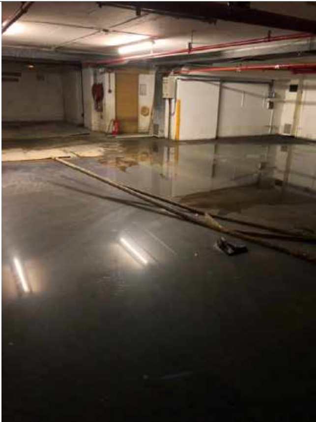
Pooled water at lowest basement point above expected sump
