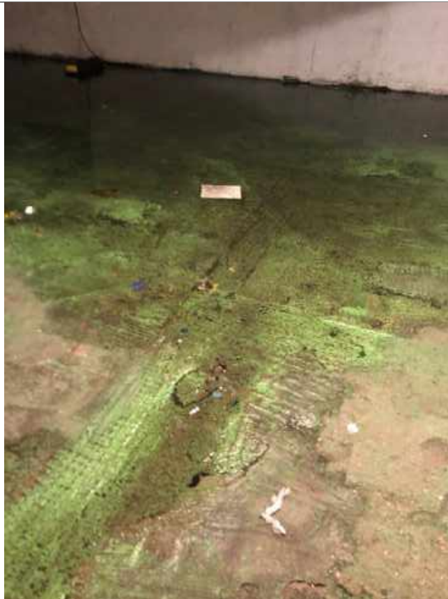
Moss growth associated with long-term dampness in sealed off basement level
