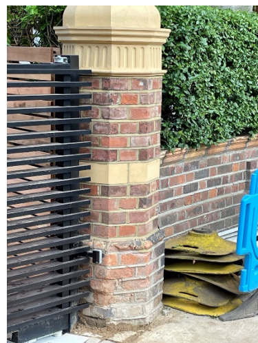
10. New terracotta & reclaimed bricks in position on No 16 pier.
