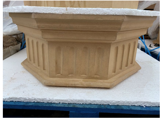
6. Intermediate capping piece, Matching exactly what was originally installed.
