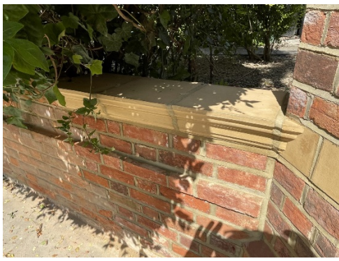
11. Wall adjacent to No18 showing replacement terracotta capping.
