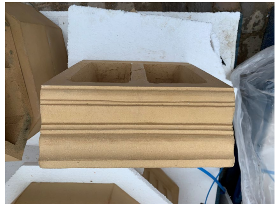
8. New wall capping piece.
