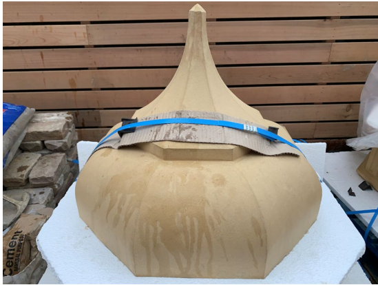
5. New capping piece, dimensioned exactly to the existing column cap.
