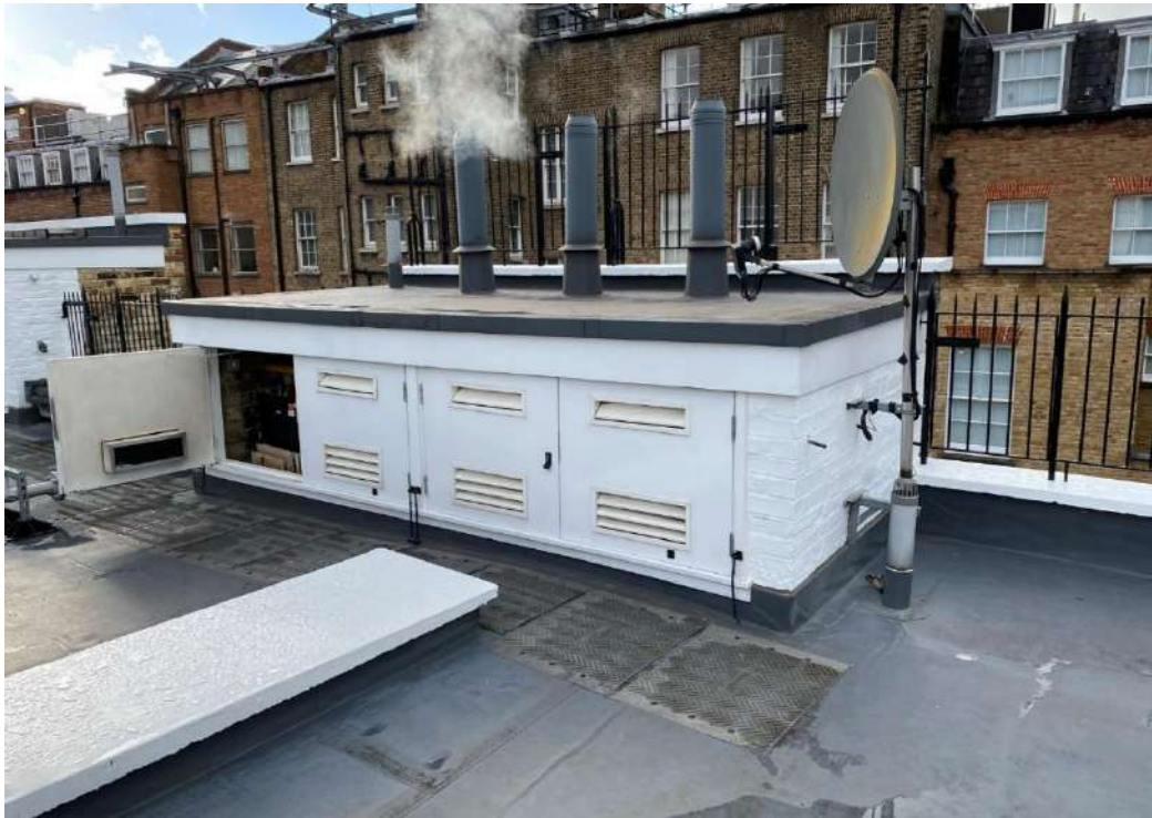
AN EXISTING PLANT ENCLOSURE AT ROOF LEVEL
