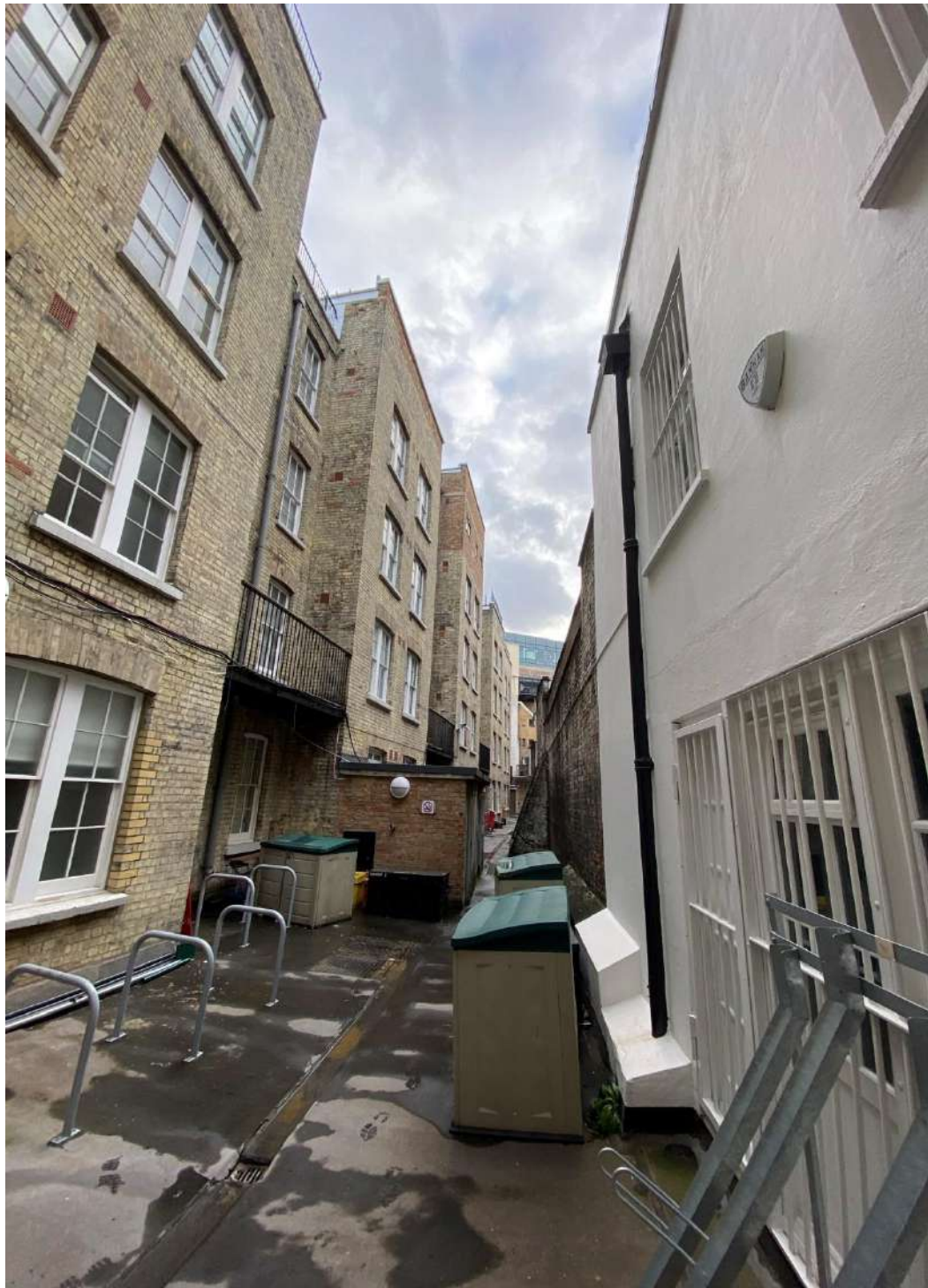
VIEW DOWN THE REAR ALLEY-WAY, LOOKING SOUTH. THE EXISTING PLANT ENCLOSURES CAN BE SEEN ATOP EACH BAY PROJECTION
