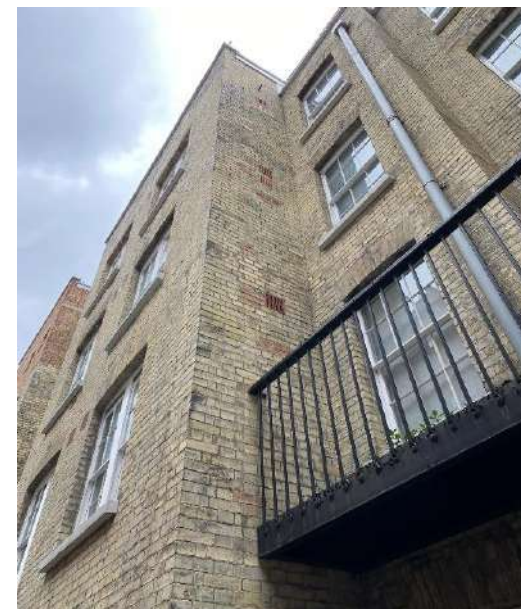
VIEW OF A TYPICAL BAY, FIRST FLOOR CAST-IRON BALCONY IN FORE-GROUND.
