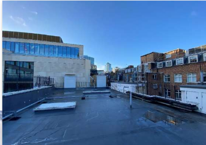
EXISTING ROOFSCAPE, LOOKING SOUTH
