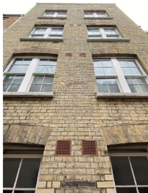
A TYPICAL REAR BAY, SHOWING THE EXISTING AIR BRICKS
