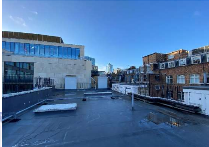
EXISTING ROOFSCAPE, LOOKING SOUTH
