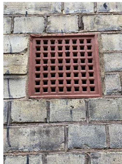
AN EXISTING TERRACOTTA AIR-BRICK
