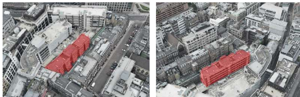
POSITION OF ST ANDREWS HOUSE ON THE CURRENT ESTATE. WORKS TO 17 CHARTERHOUSE STREET SEEN UNDERWAY.
