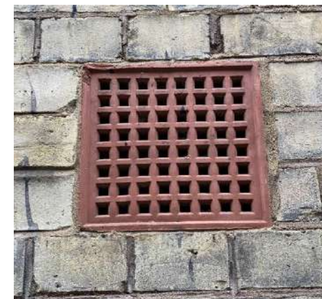
AN EXISTING TERRACOTTA AIR-BRICK
