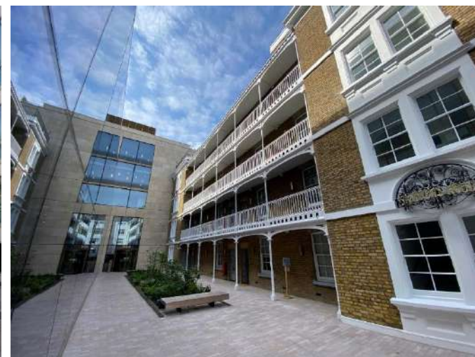
VIEW OF FRONT (EAST) LOOKING SOUTH
