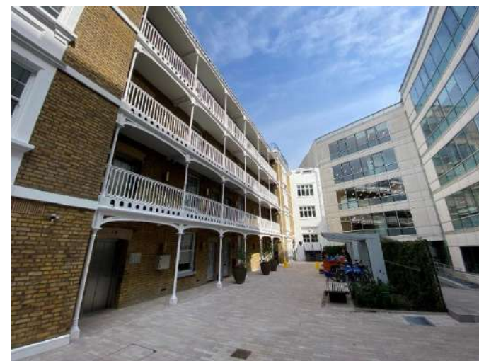
VIEW OF FRONT (EAST) LOOKING NORTH
