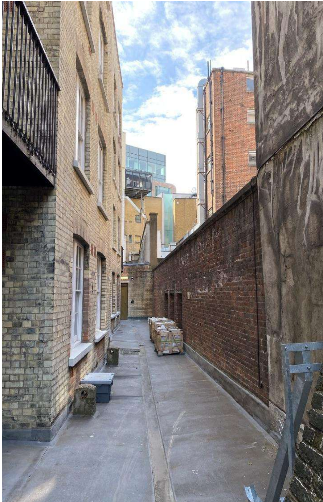
VIEW DOWN THE REAR ALLEY-WAY, LOOKING SOUTH
