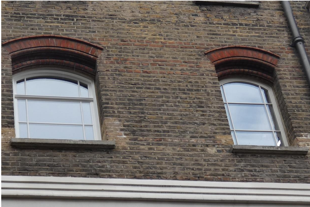
Replaced and existing casement windows
