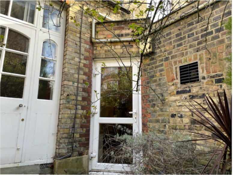
External doors to garden from living and dining rooms showing 510mm change in floor level between the two rooms.
