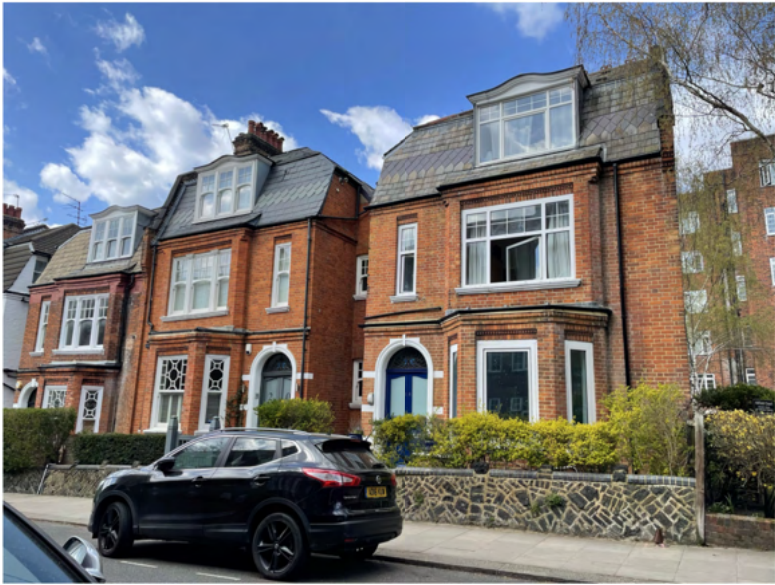
Front elevation No. 18 Glenloch Road (end of terrace) - burnt lava bricks and slate mansard roof
