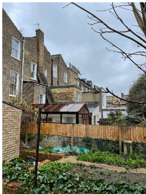
View of the rear garden of No 61 and the new extensions at the back of No 59 and No 57
