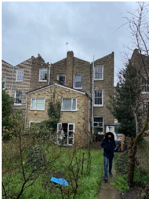
View of the existing rear elevation of No 63, with No 65 being visible to the far left
