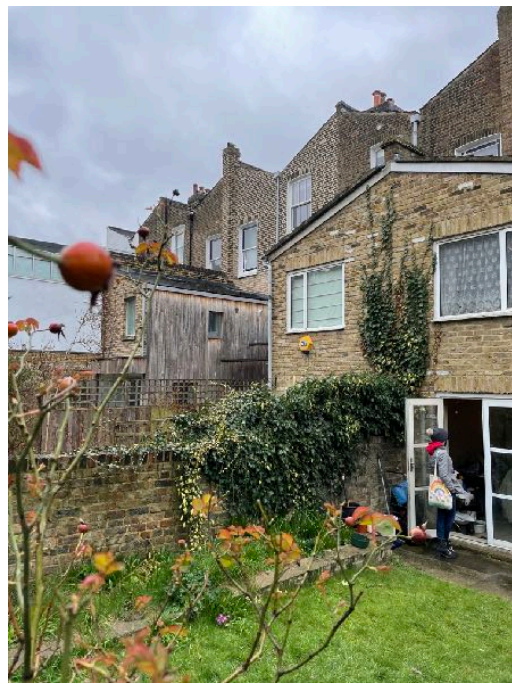
View of the rear facade of No 63, with the boundary wall and mirror image' rear part of No 65 in the background
