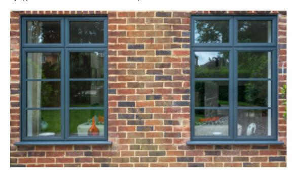
• Any new windows within 800mm of finished floor level, and doors and sidelights within 300mm will need to be fitted with safety glass to BS6206.
