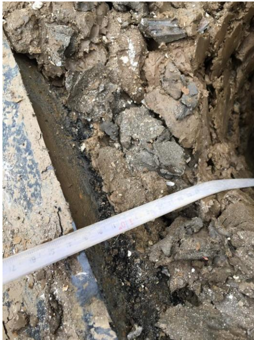
Plate 7 - TAPE MEASURE CONFIRMING BOREHOLE DEPTH AT 10M
