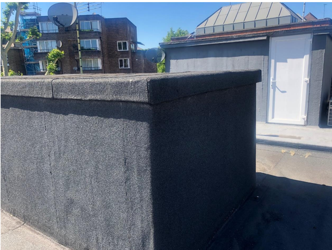
6. 25 Crossfield Road roof looking towards 24 Crossfield Road roof structure.
