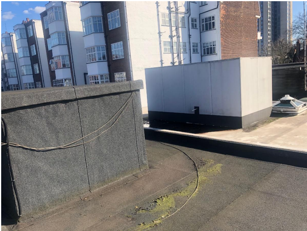
4. Existing roof huts at 25 and 26 Crossfield Road
