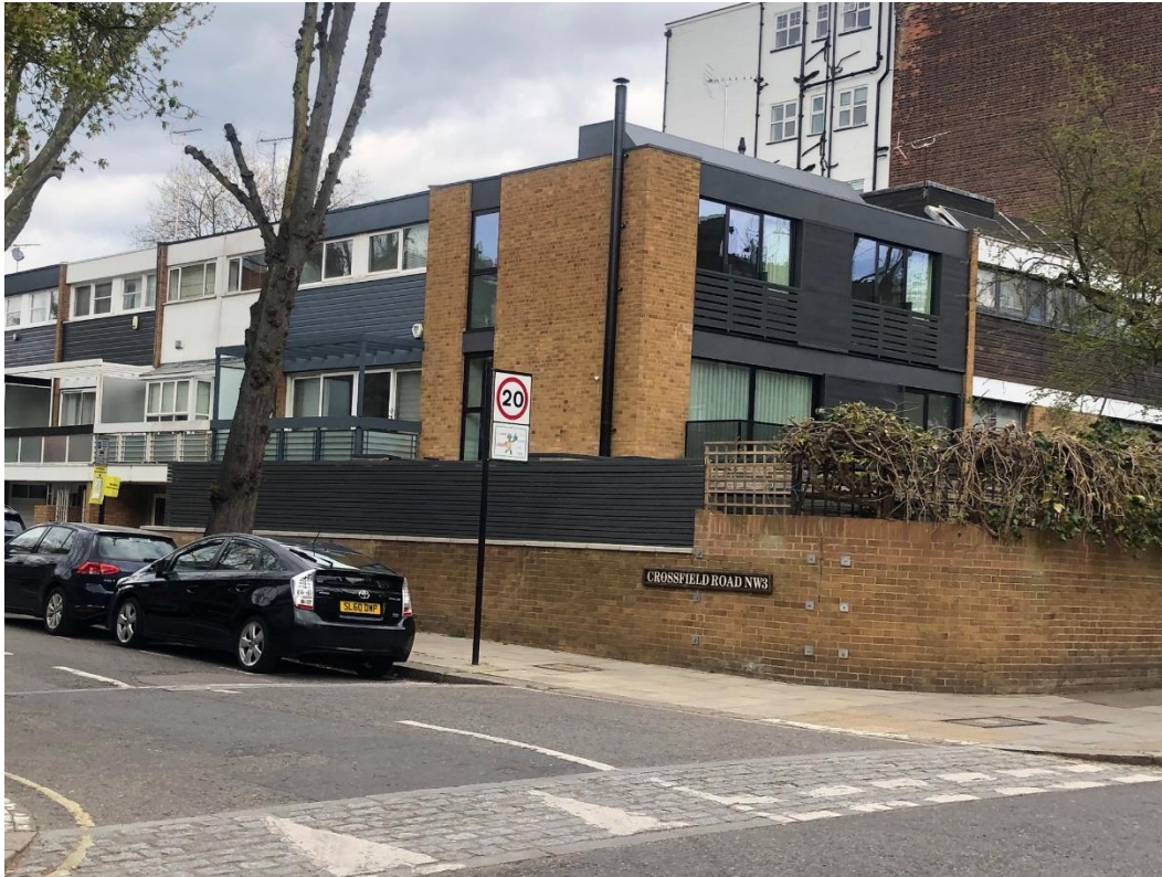
3. Corner of Crossfield Rd and Eton Ave with 52 & 50 Eton Ave solar panel installations
