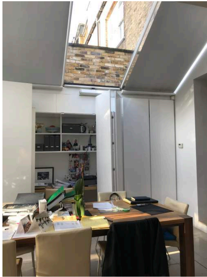
PHOTO 12: Interior view of dining room to 3/18 Aberdare Gardens with fully glazed pitched roof.
