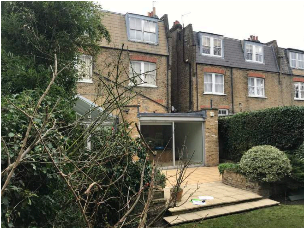
PHOTO 07: Rear elevation of 18 Aberdare Gardens showing part ground floor flat (flat 3/18) with No. 20 on RHS.
