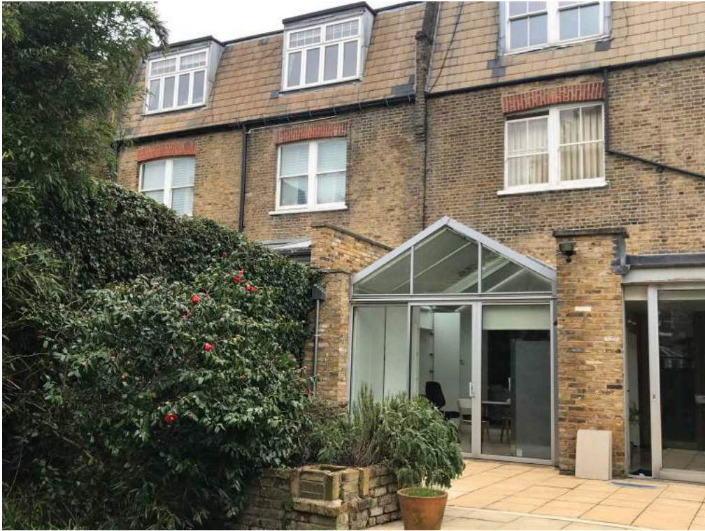
PHOTO 06: Rear elevation of 18 Aberdare Gardens showing part ground floor flat (flat 3/18) with No. 16 on LHS.
