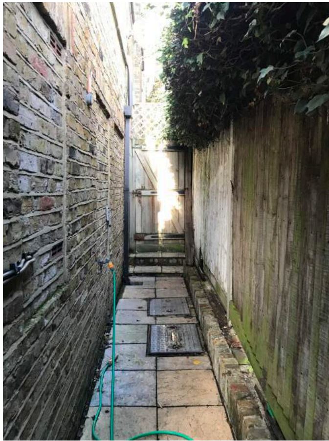
PHOTO 08: Side passage to 18 Aberdare Gardens looking towards the street entrance.
