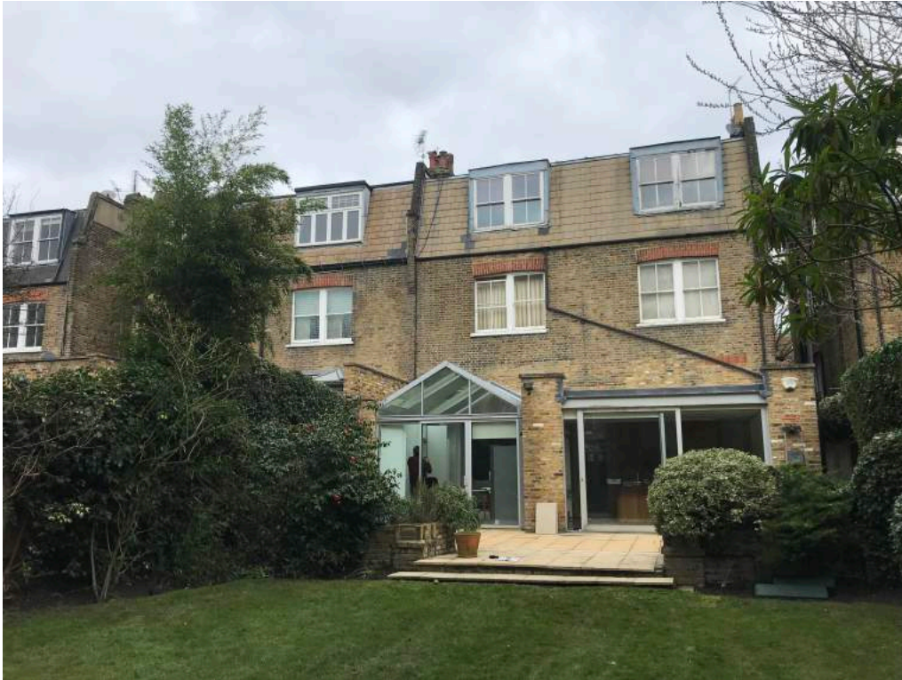
PHOTO 01: Rear elevation 18 Aberdare Gardens with Flat 3 at ground level.
