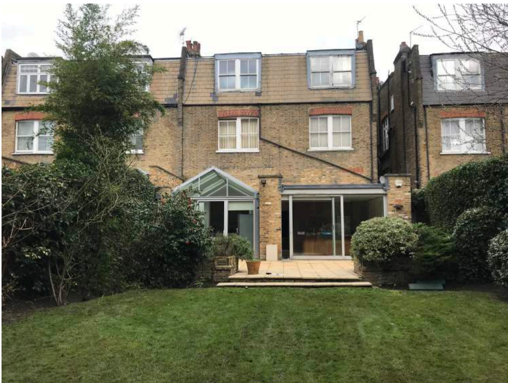
PHOTO 05: Rear elevation of 18 Aberdare Gardens with No. 16 on LHS and No. 20 on RHS.
