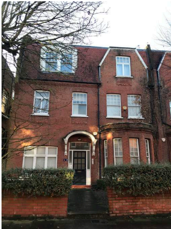
PHOTO 03: Front elevation of 18 Aberdare Gardens with flat No. 3 at ground level.
