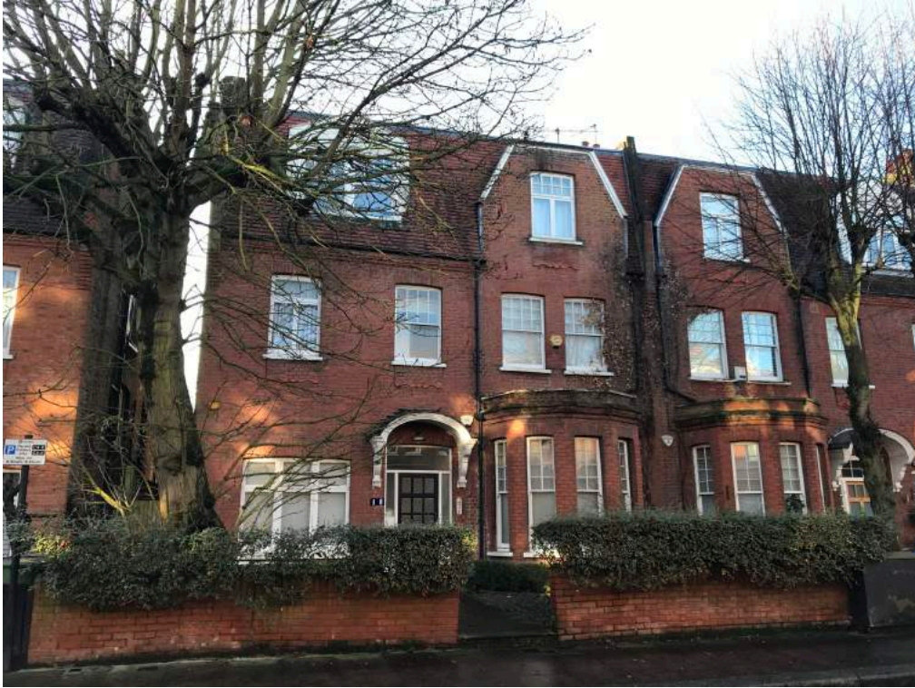
PHOTO 02: Street/ front elevation of 18 Aberdare Gardens with No. 20 on LHS and No. 16 on RHS.
