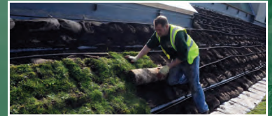
■ Turf laying in progress
